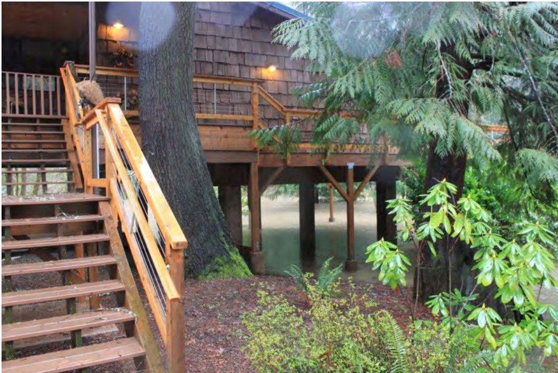
Mitigation Success - Abernethy Creek elevation completed in March 2010 and successfully tested on January 19, 2012. Source: Clackamas County
