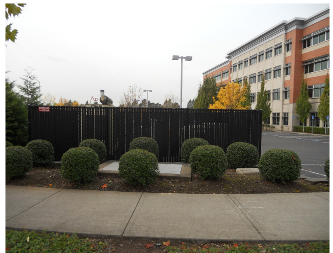
PSB generator equipment screening from Kaen Road Slatted painted chain link, 6-foot high.
