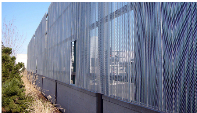
Central Utility Plant Equipment Enclosure Fence: Split face CMU with metal panels
