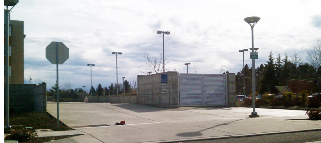
Louvered fence at DSB transformer, Library Court Fence: Concrete and louvered metal panel, 12-foot high. Concrete and Metal panel
