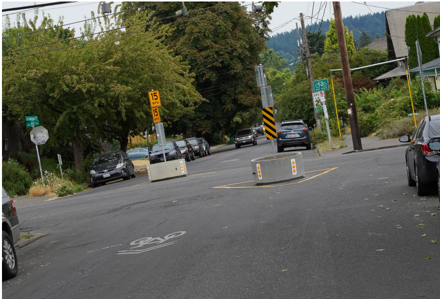
Concrete planters and 15 mph advisory signs at SE Salmon St & SE 20 th Ave. Photo source: Bike Portland
