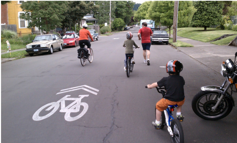
Sharrows marking along a neighborhood greenway in Portland, OR. Photo source: Nelson\Nygaard
