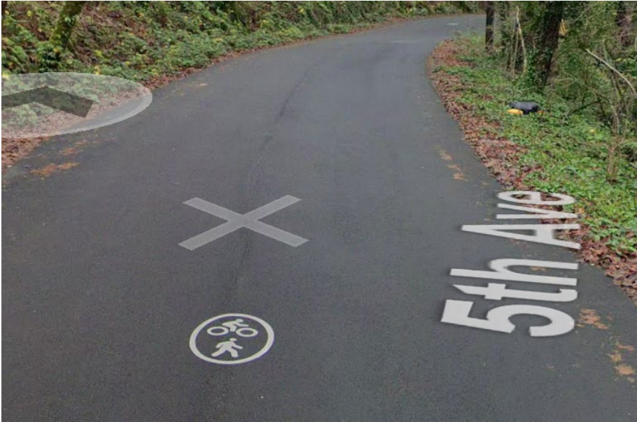
Shared pedestrian and bicycle pavement marking on 5 th Avenue in Oregon City. Image source: Google Streetview
