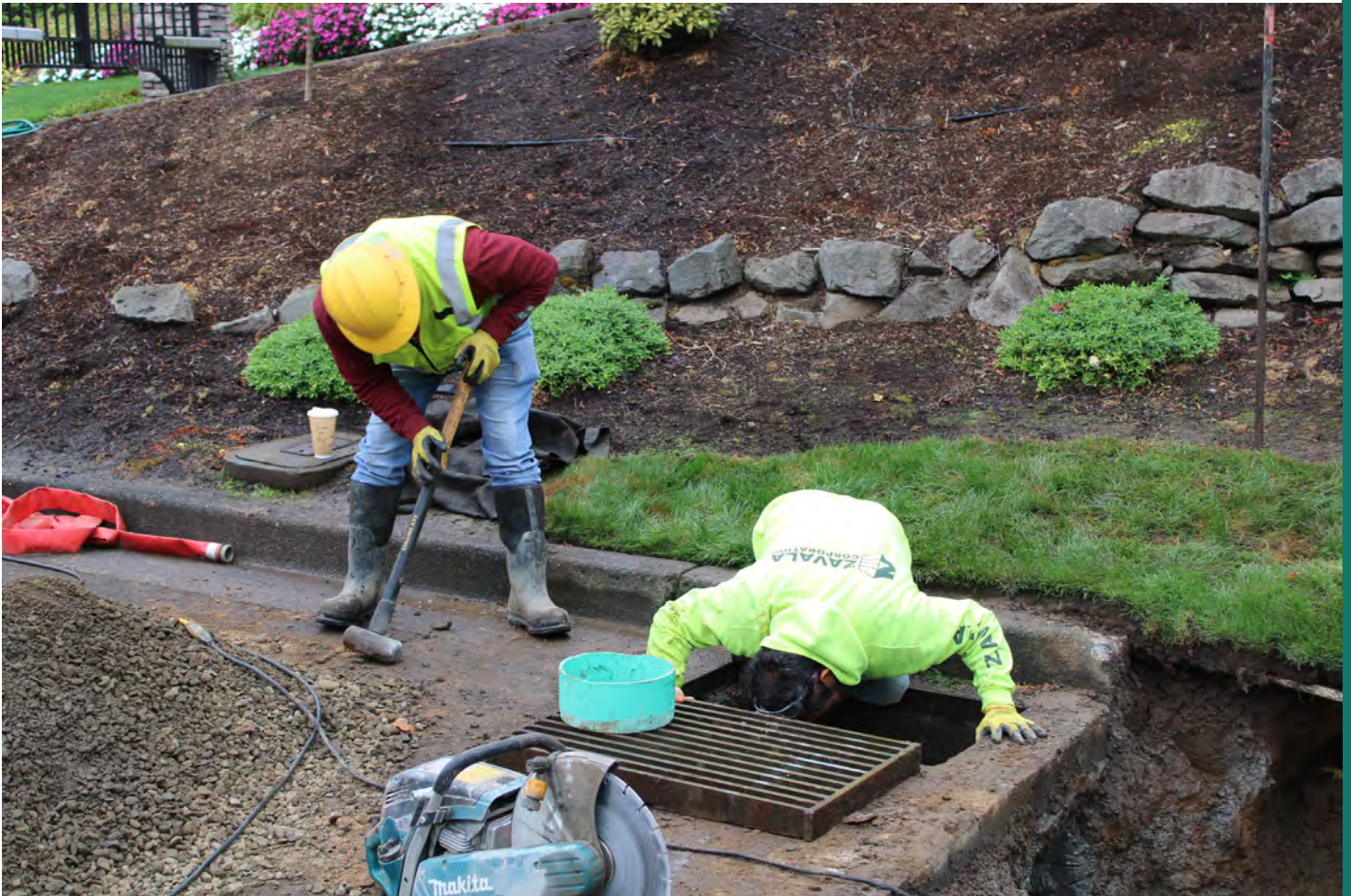
Repairs to a stormwater drain
