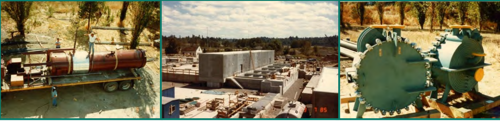
Photos from construction of the Tri-City WRRF in the 1980's
