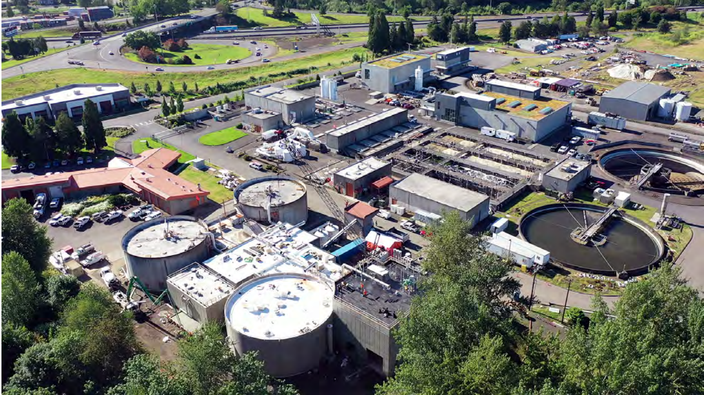
Tri-City Water Resource Recovery Facility
