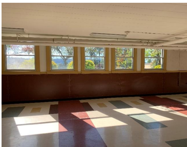
Cafeteria, looking west
