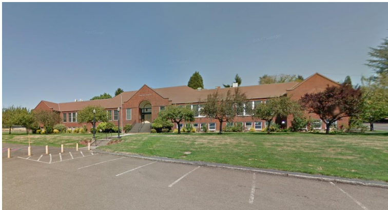
Concord School, west façade
