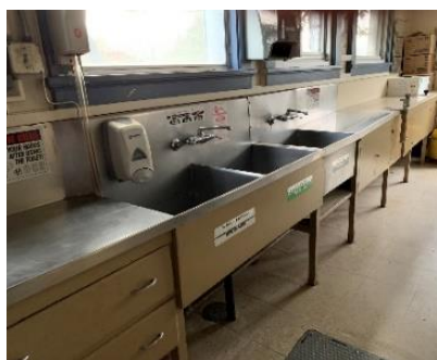
Kitchen, sink/counter, south wall
