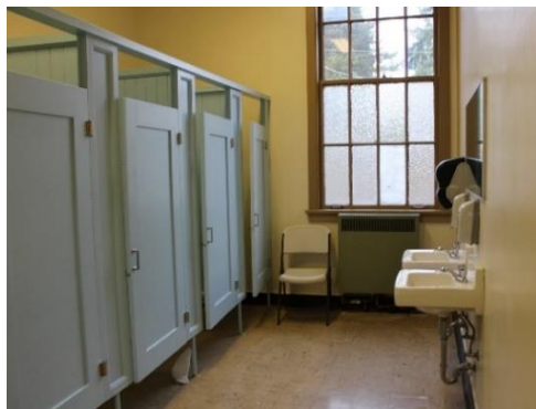
Original 1936 girl's restroom, upper level
