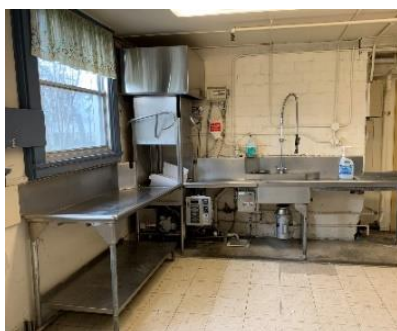
Dishwashing area, kitchen, NW corner
