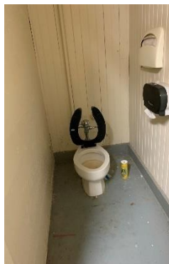
Original boy's restroom, locker area, lower level
