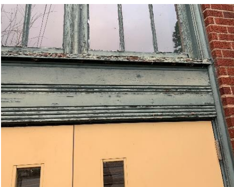
Original wood transom windows, south facade
