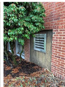
Louver/panel, south facade
