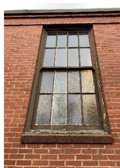
Original wood window, girl's restroom
