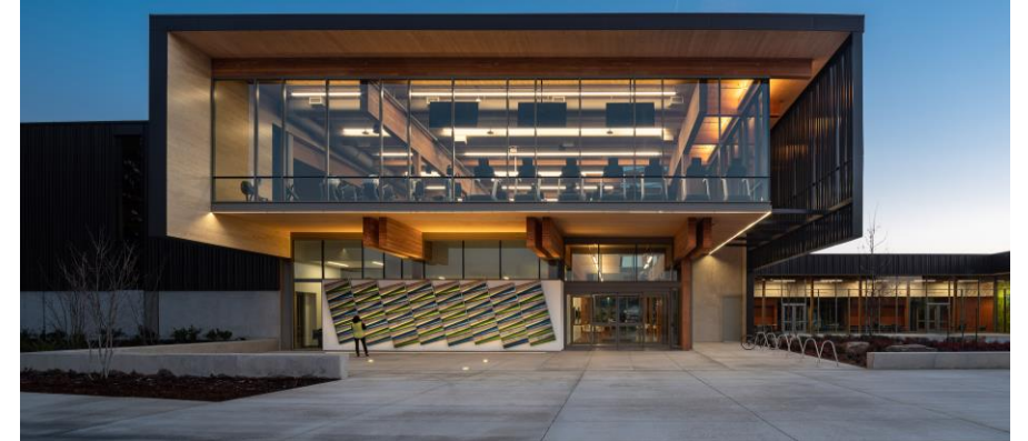
Integrated into building exterior at Hidden Creek Community Center
