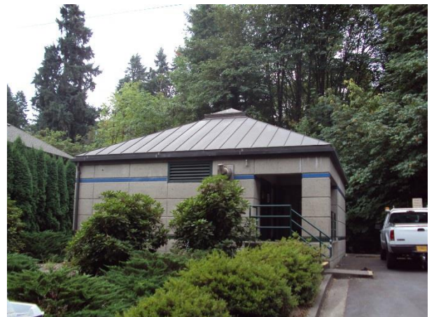
WES Telemetry System Replacement
