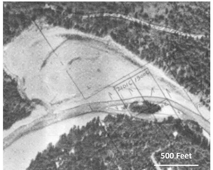
D. Aug 1965 - Post USACE levee completion Corps channelization and survey lines for future development.
