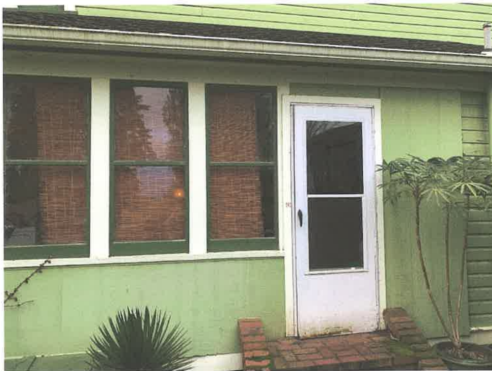
Detail of east (rear) addition. T111 plywood siding, non-period door + casework & non-original storm windows
