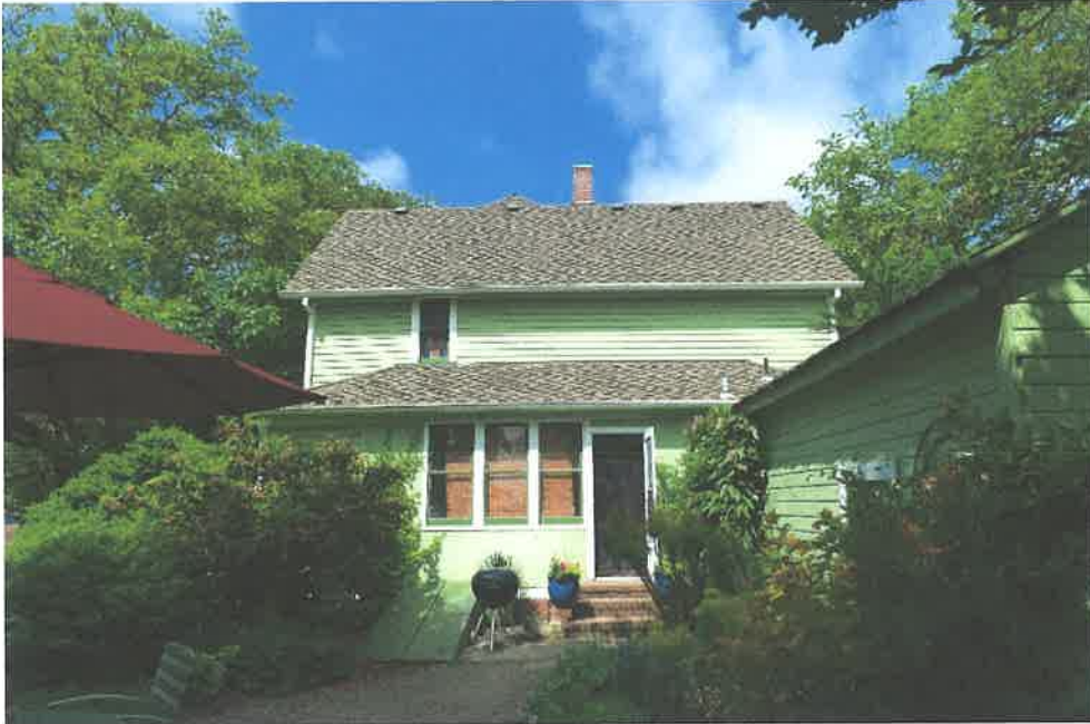
Existing east (rear) façade (non-original hipped-roof addition)
