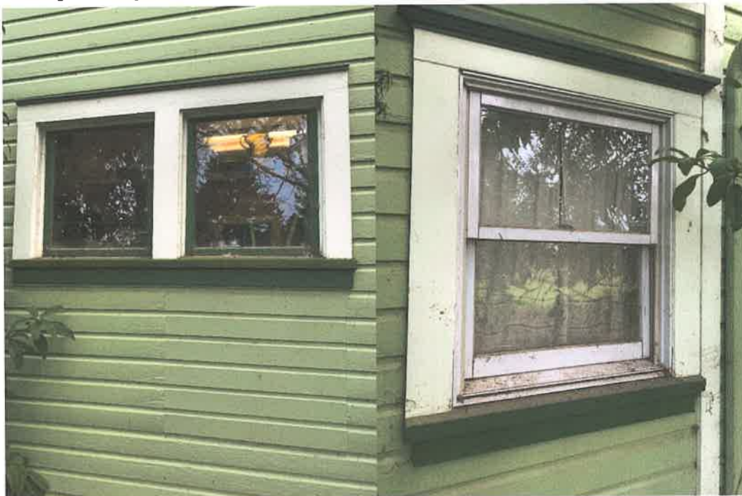
Detail of non-original kitchen windows and cut siding below. Detail of non-original bathroom window
