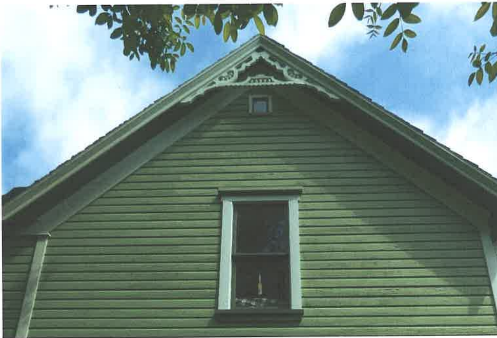
Existing gable trim & ornamentation (shown at south gable) To be replicated in the proposed east dormer
