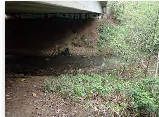
Stream below Sunnyside Bridge looking west with blackberry
