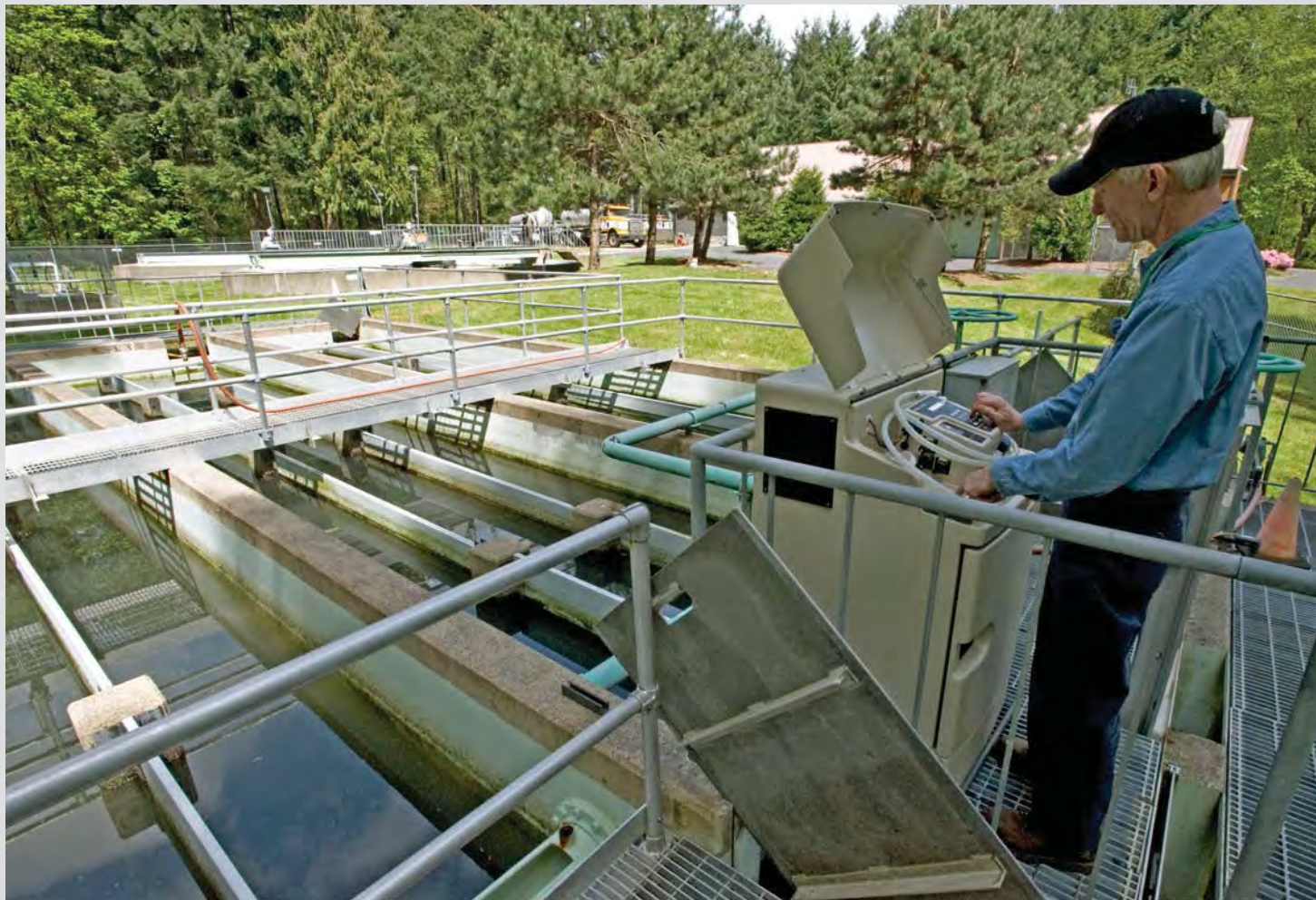
One of WES' Wastewater Plant Operators performs sampling of the effluent in the chlorine contact basin at the Hoodland Water Resource Recovery Facility in Welches, OR
