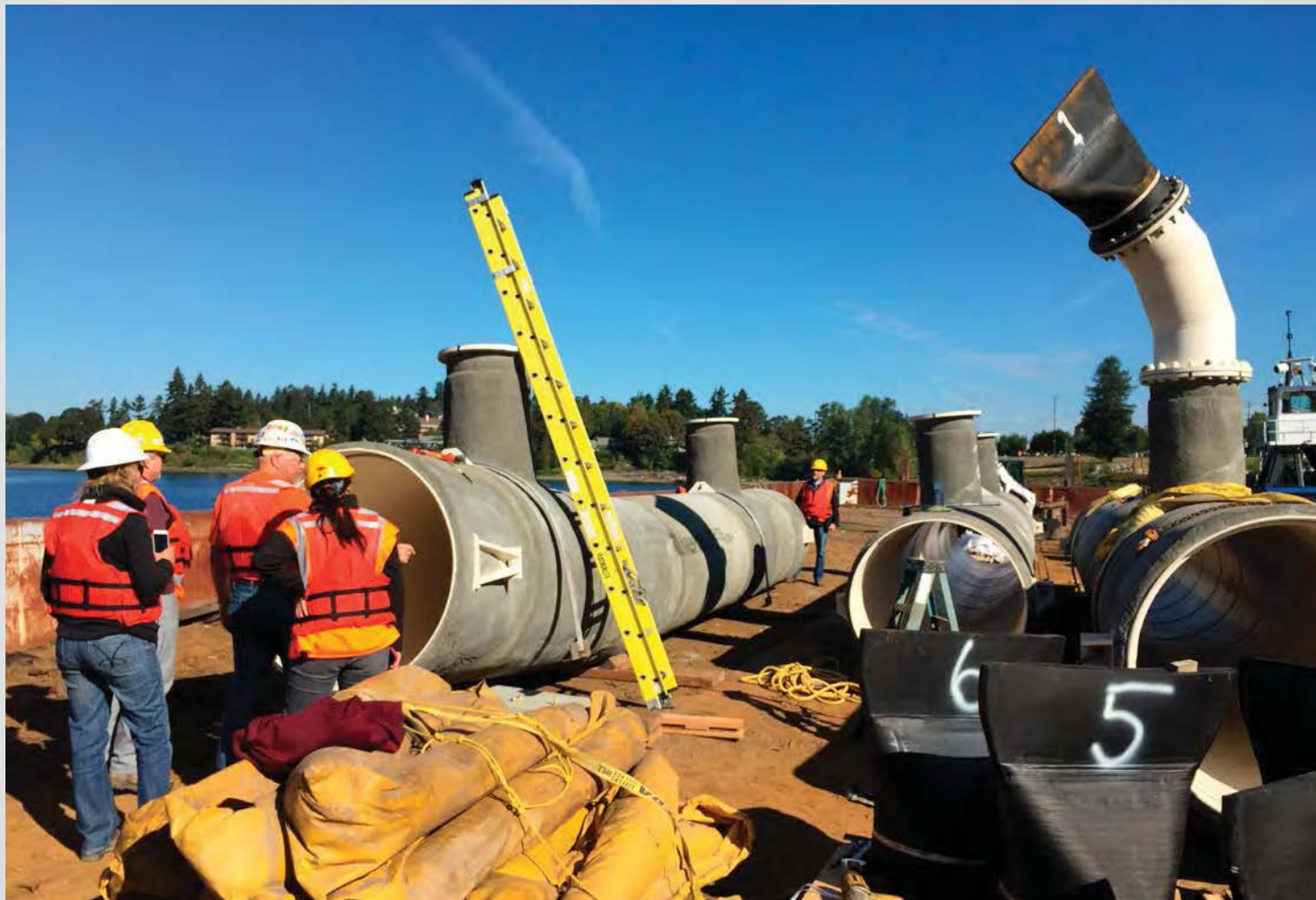
Crews work on replacing the outfall pipe at Kellogg Water Resource Recovery Facility in Milwaukie, OR
