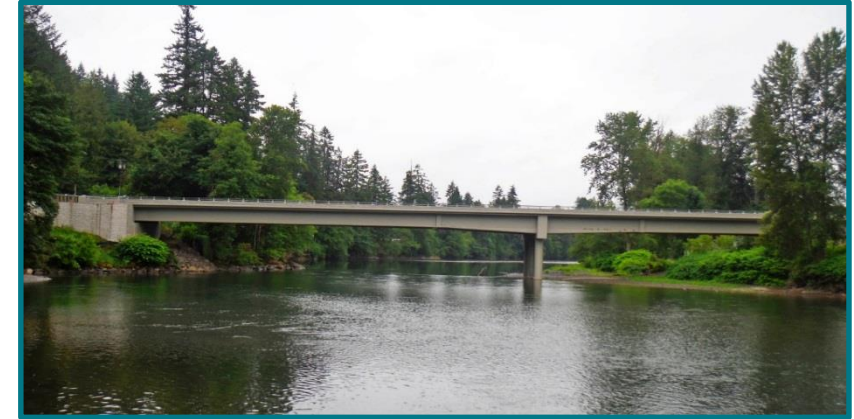
Carver Bridge Over the Clackamas River
