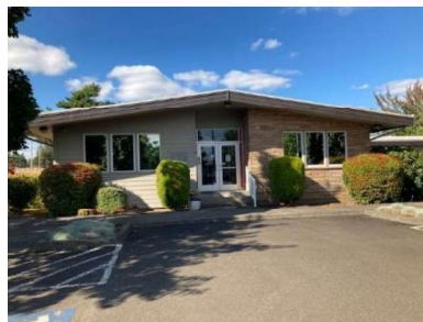
#5 Technology Services 121 Library Ct. Ore. City
