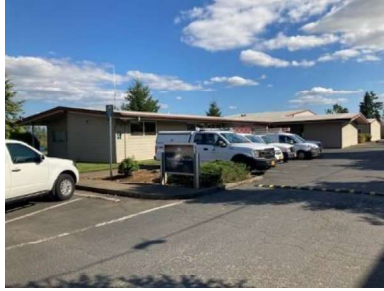
#8 Telecom Services 168 Warner Milne Rd. Ore. City
