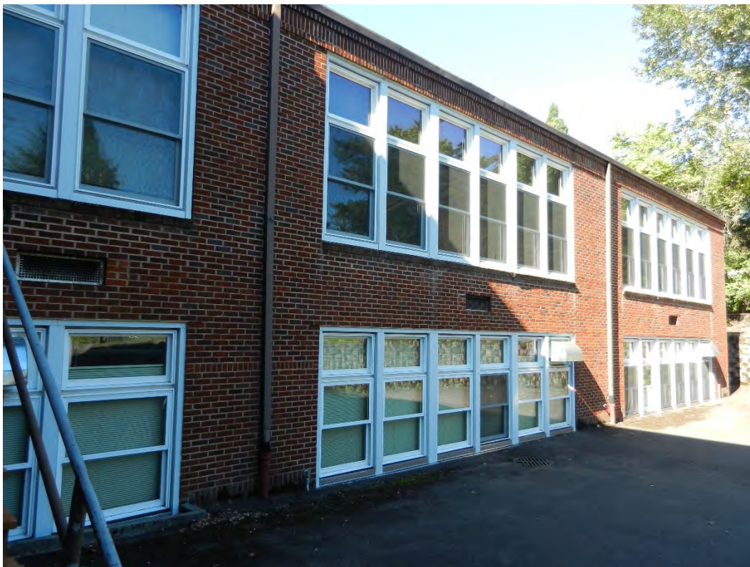
Southern façade of rear wing addition, camera facing northeast (ARG, October 2019).
