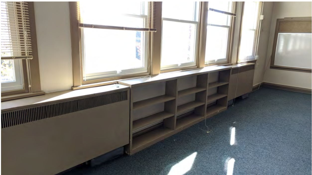
Representative view of built-ins in upper-floor classroom in 1936 building (ARG, October 2019).
