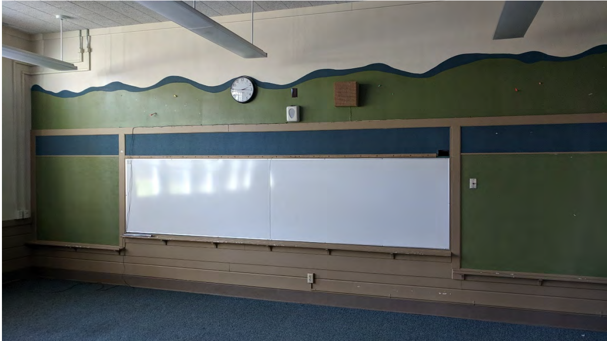
Representative view of chalkboard surrounds in classroom in 1948 addition (ARG, October 2019).
