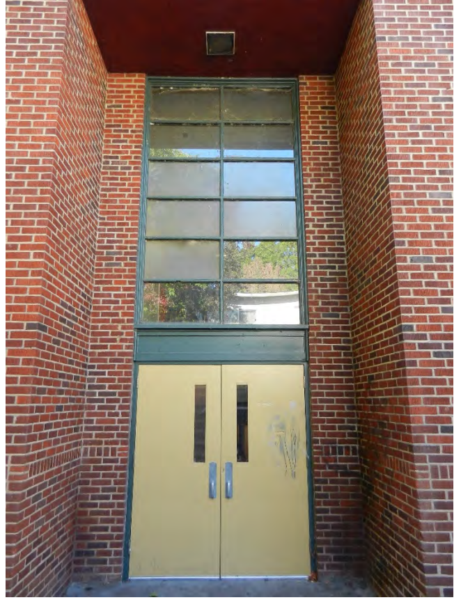
Eastern façade of rear wing addition, camera facing west (ARG, October 2019).
