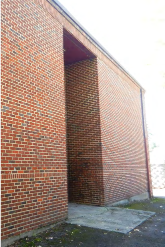
Eastern façade of rear wing addition, camera facing northwest (ARG, October 2019).
