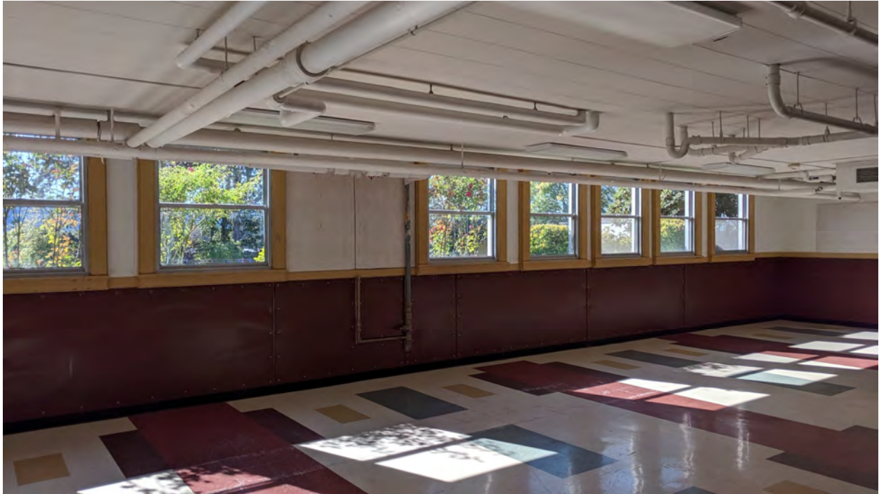
Cafeteria in basement of 1936 building (ARG, October 2019).
