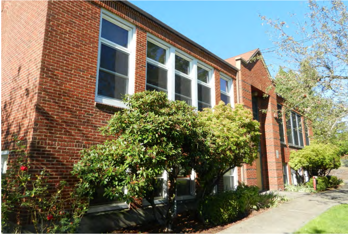
Southern façade, camera facing northeast (ARG, October 2019).
