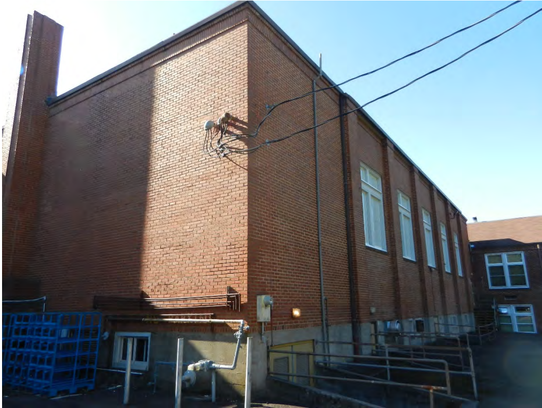
Rear (eastern) façade, camera facing northwest (ARG, October 2019).
