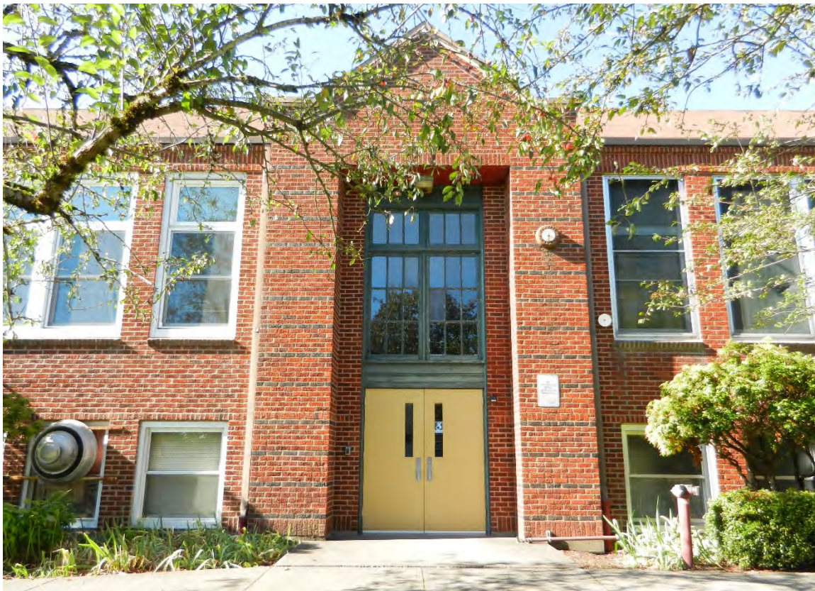
Southern façade, camera facing north (ARG, October 2019).
