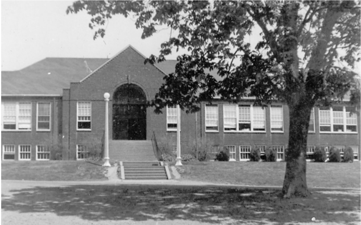
Figure 3. Photograph showing western façade of Concord School building, 1955. Note multilight wood windows and lampposts (Oak Lodge History Detectives).
