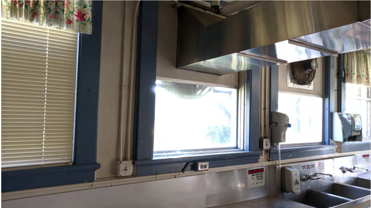
Window casings in kitchen in basement of 1936 building (ARG, October 2019).
