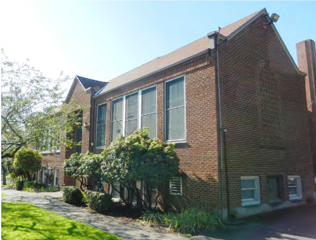
Southern façade, camera facing northwest (ARG, October 2019).
