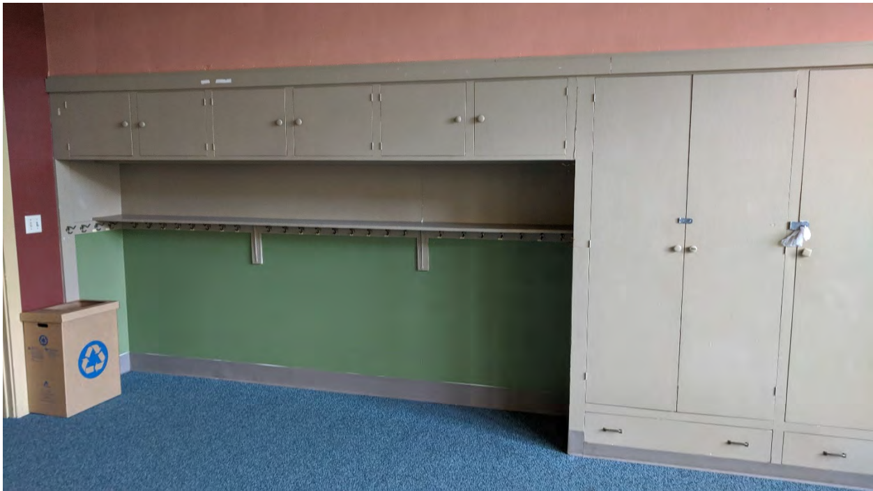
Representative view of built-ins in classroom in 1948 addition (ARG, October 2019).
