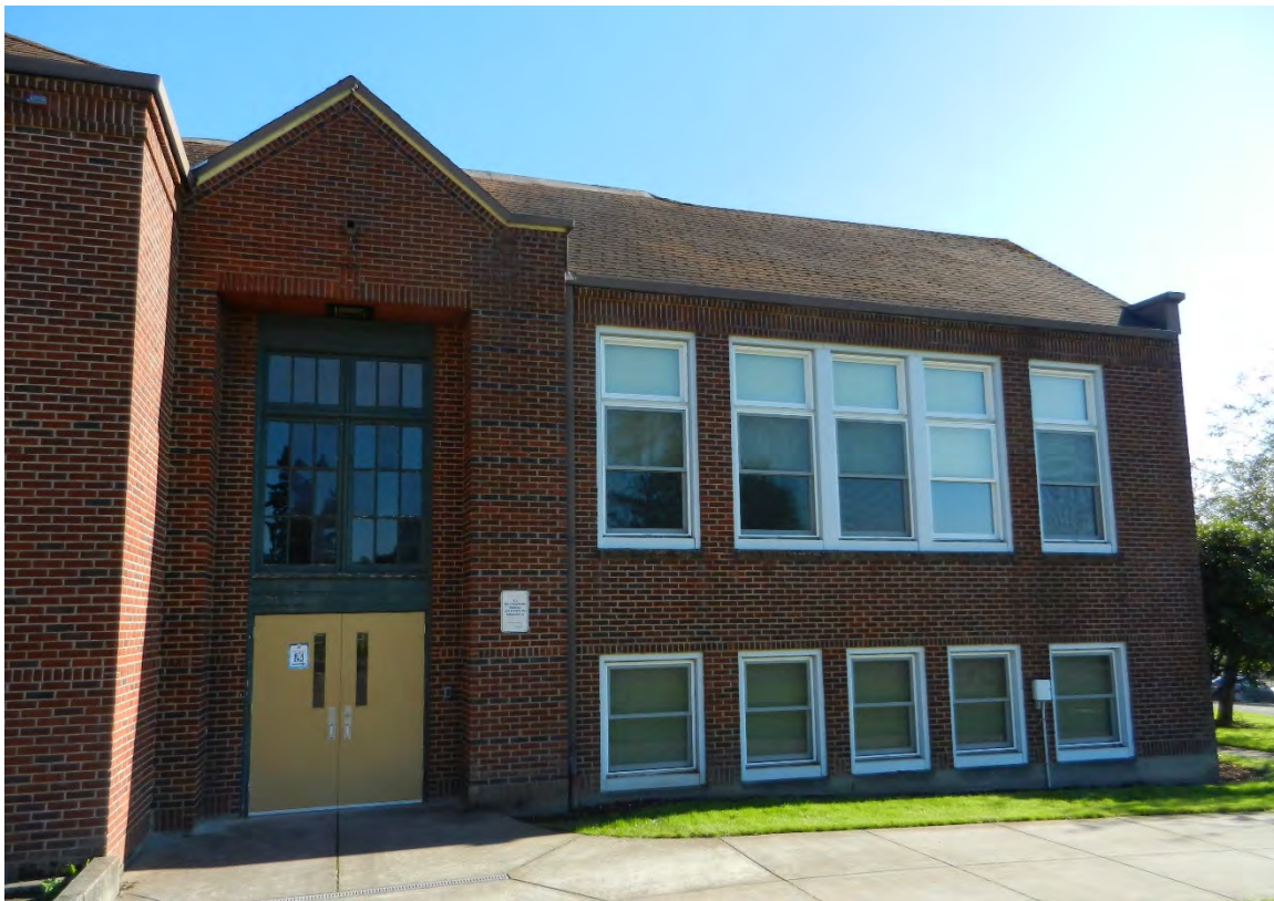
Northern façade, camera facing south (ARG, October 2019).
