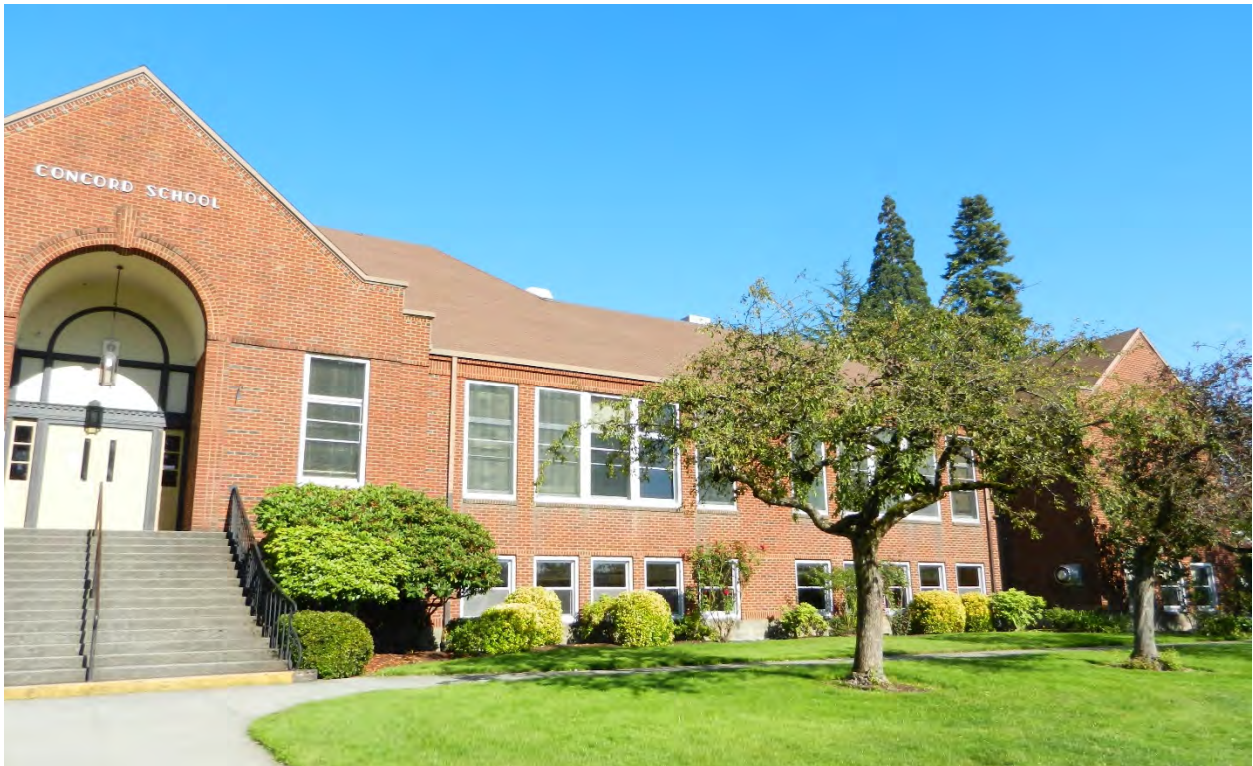
Southern portion of primary (western) façade, camera facing east-southeast (ARG, October 2019).
