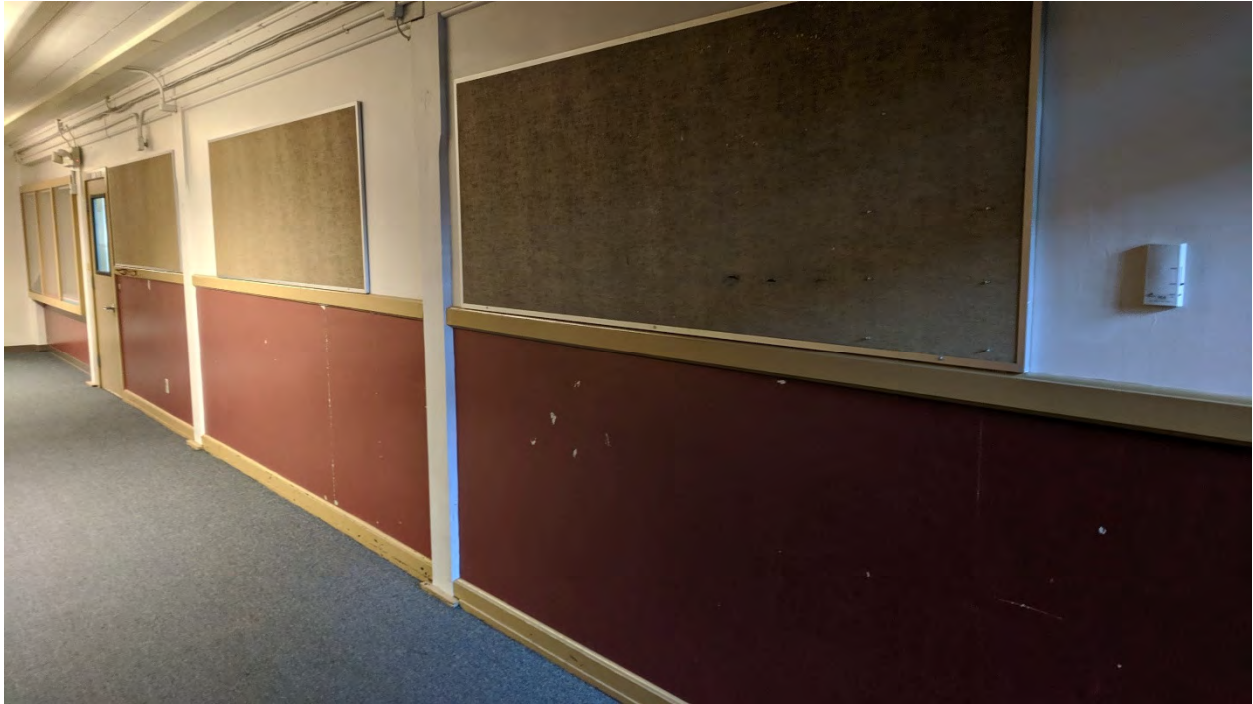
Representative view of corridor in 1948 addition (ARG, October 2019).
