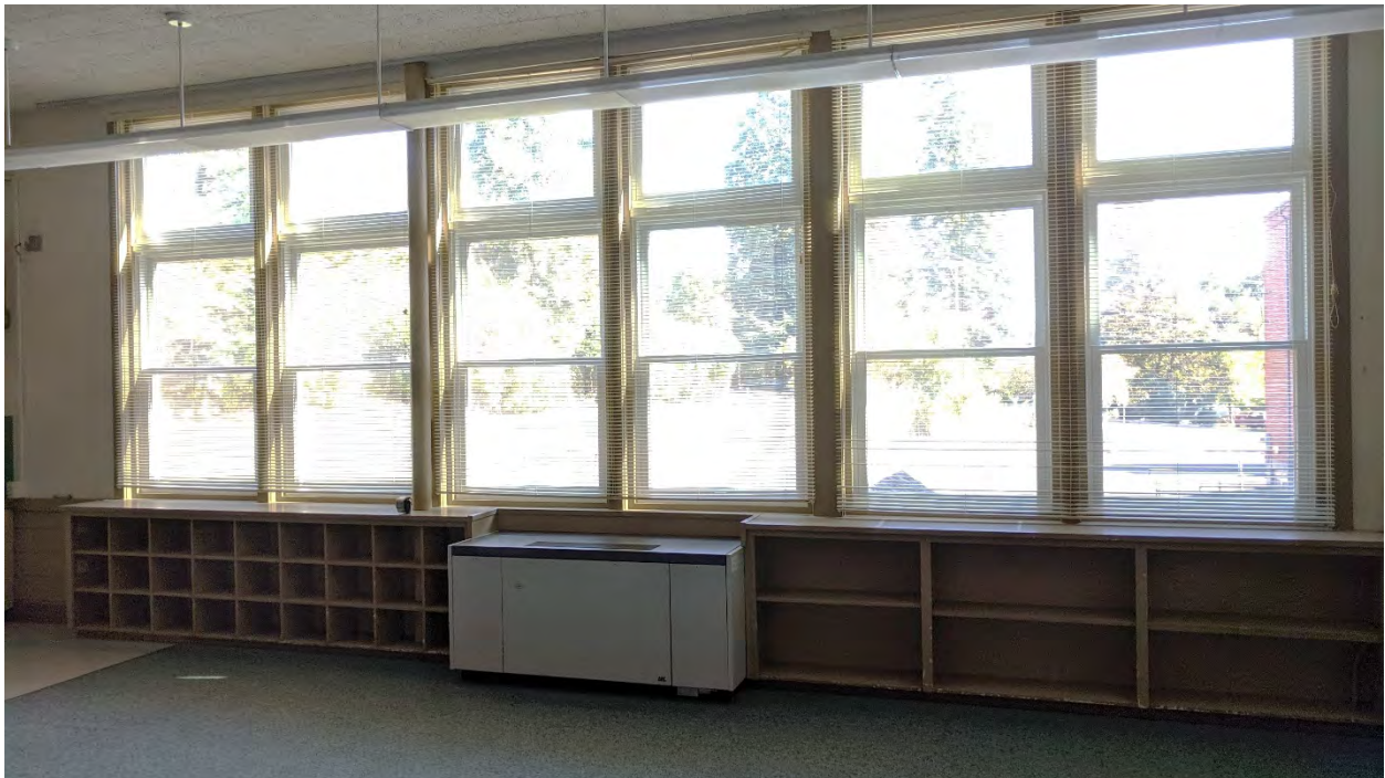
Representative view of built-ins in upper-floor classroom in 1948 addition (ARG, October 2019).
