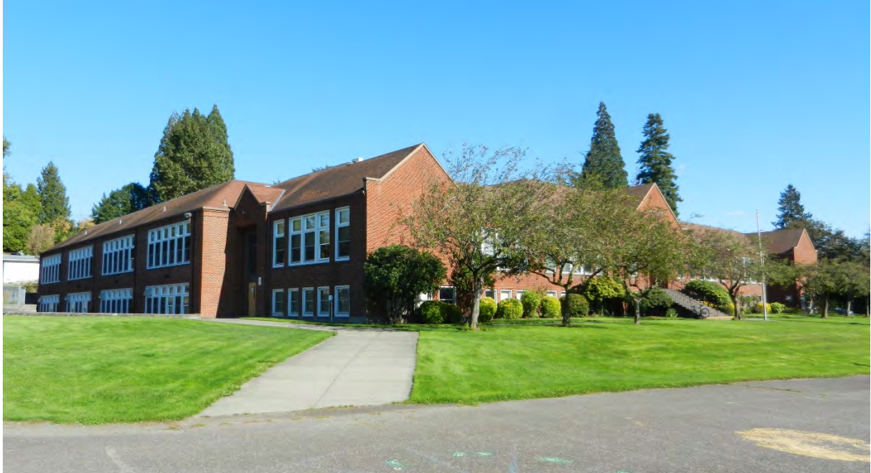
Lateral view of the Concord School showing the primary (western) façade of the 1936 building (right) and the 1948 addition (left), camera facing southeast (ARG, October 2019).
