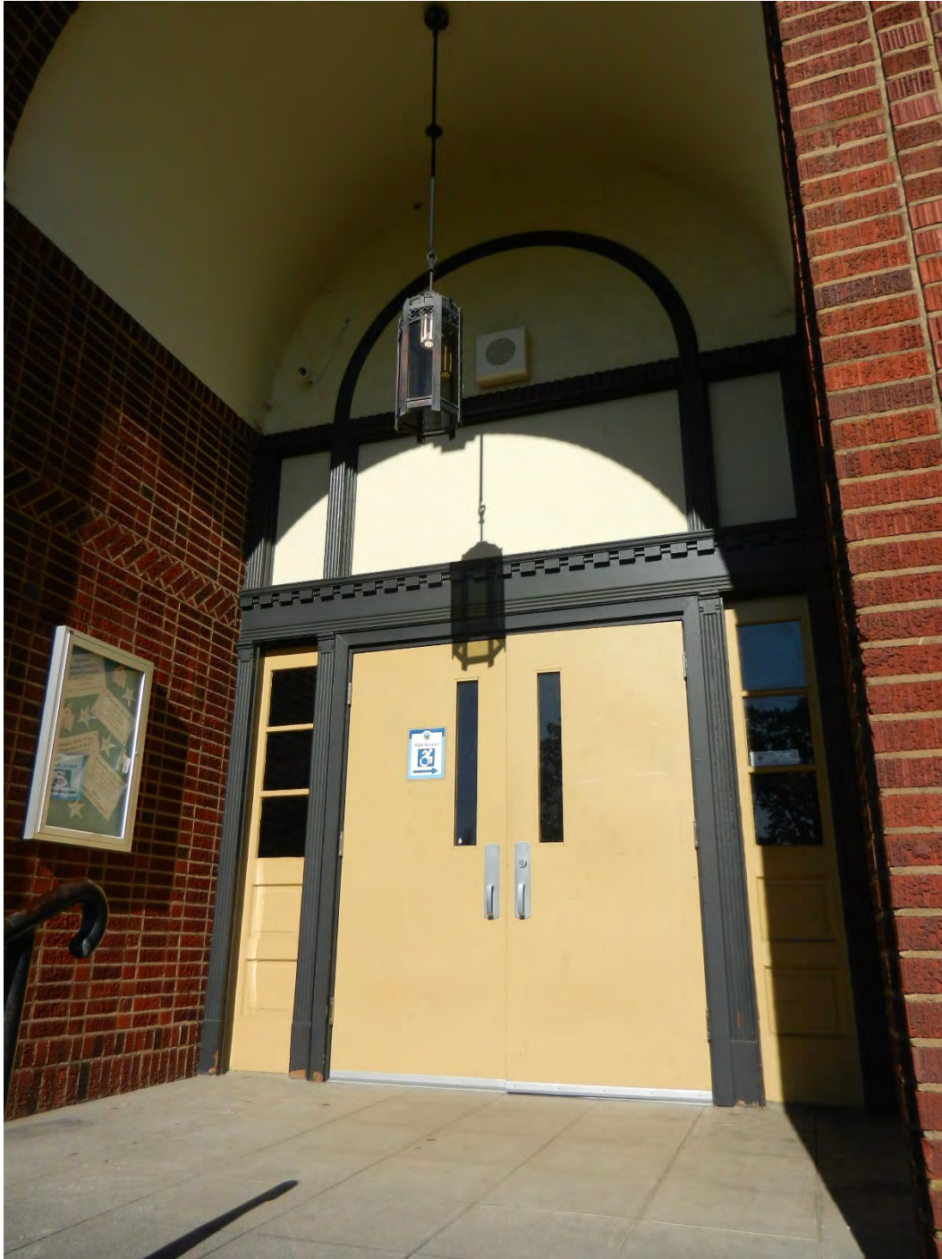
Primary entrance, western façade, camera facing east-northeast (ARG, October 2019).
