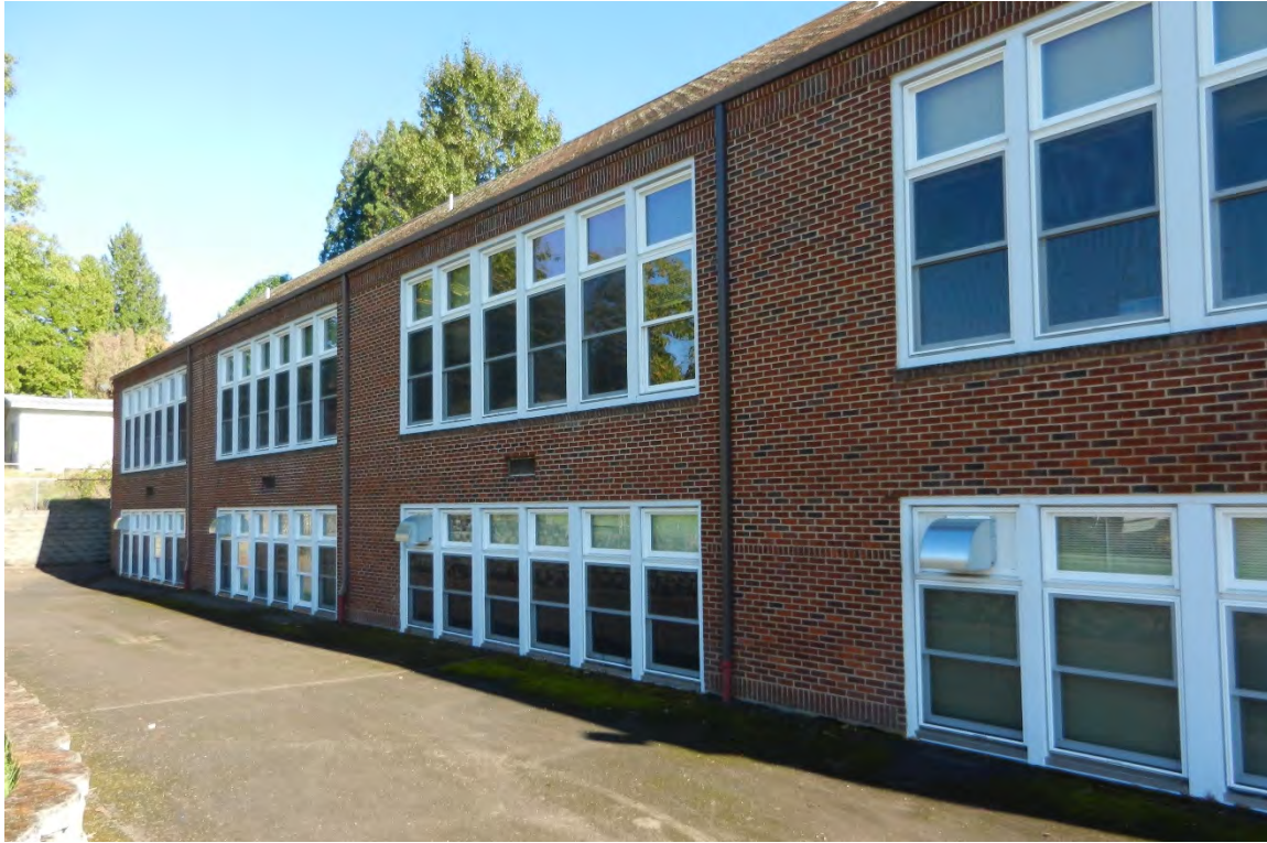
Northern façade of rear wing addition, camera facing southeast (ARG, October 2019).
