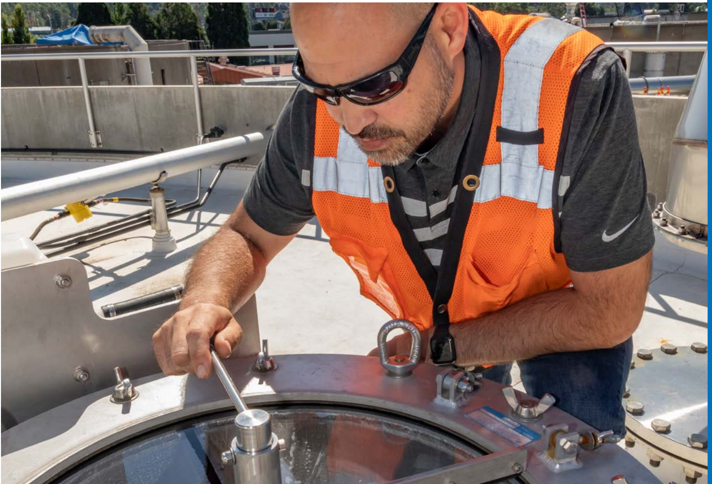
Viewing the new digester through the top porthole
