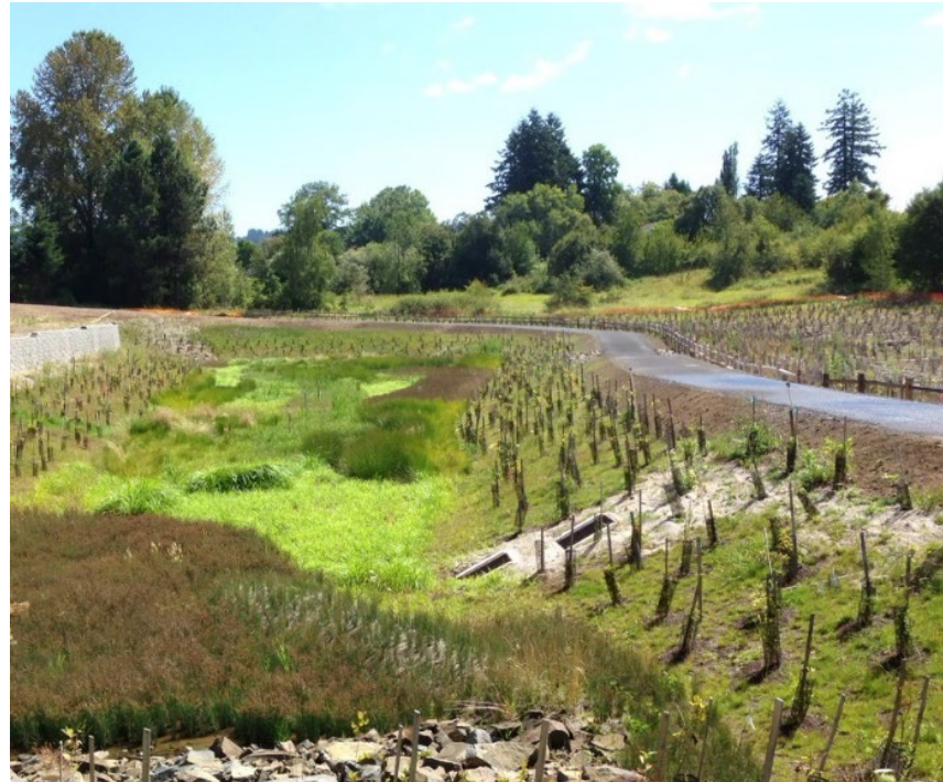
Regional stormwater facility; North Bethany in Washington County
