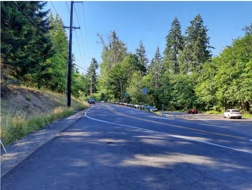
Photo 3. Overview of the project APE at the intersection of SW Stafford Road and SW Johnson Road. The view is towards the south-southeast.
