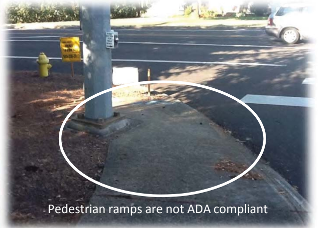
Utility pole located in pedestrian ramp – NE corner
