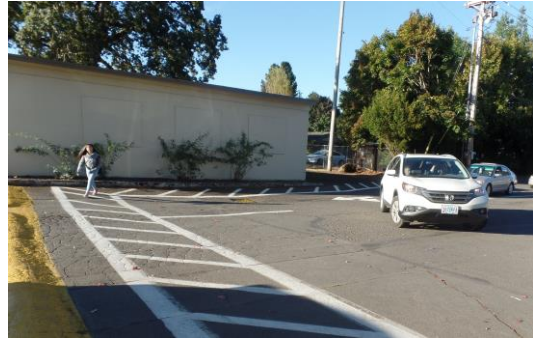
Striped shoulder and crosswalk provide access to student approaching the school on Hood St.
