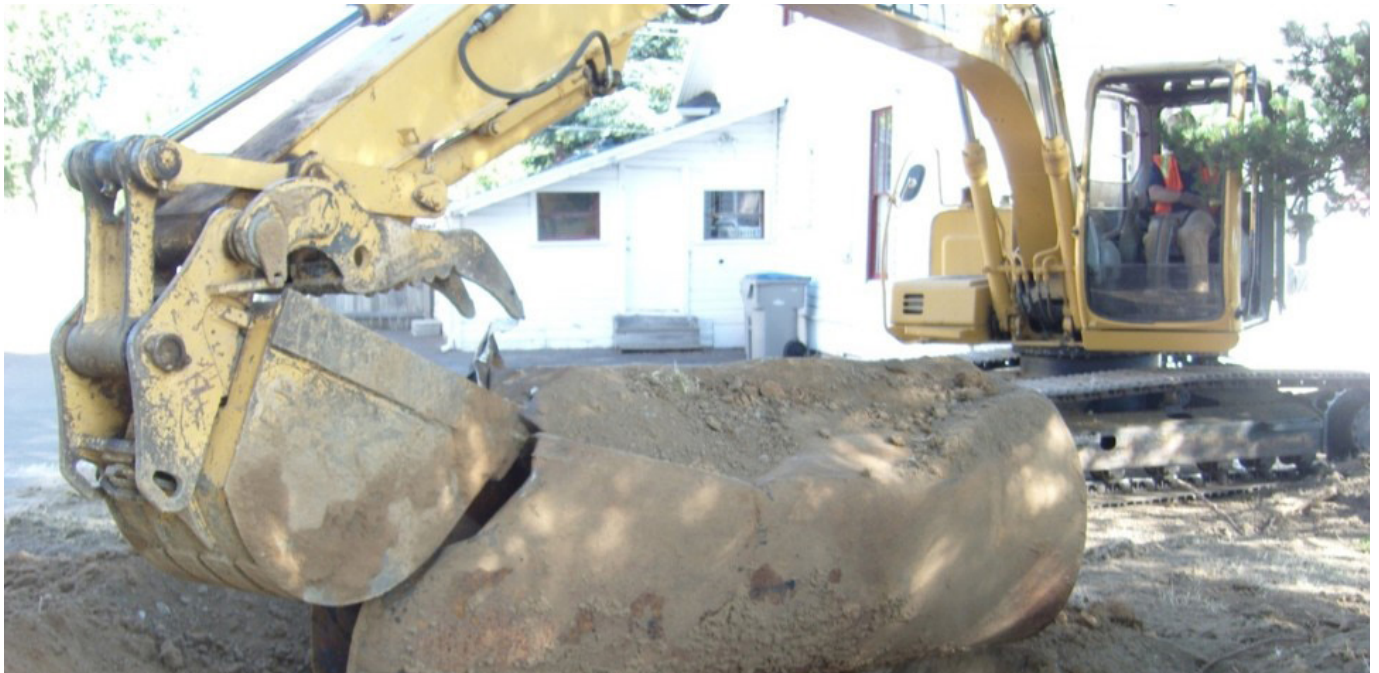
Image 2: A tank being decommissioned before redevelopment
