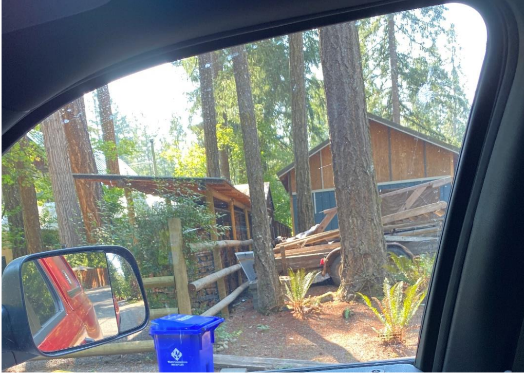
Figure 2 - Subject structure and its proximity to neighboring buildings
