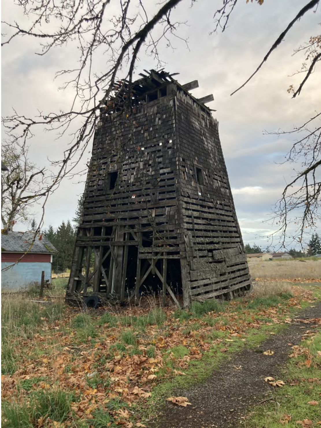
WATER TOWER (Front)
