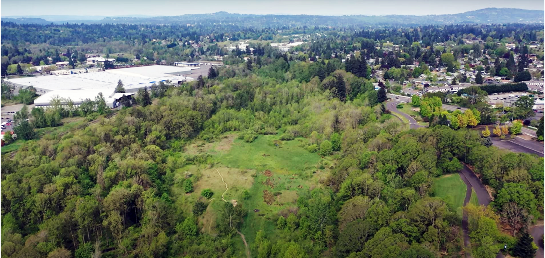
Aerial view looking west
