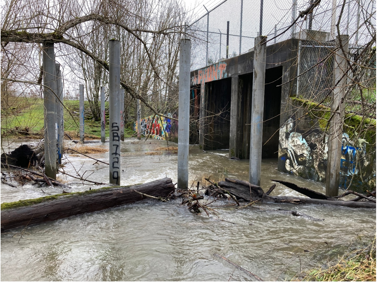
View of upstream end of water control structure
