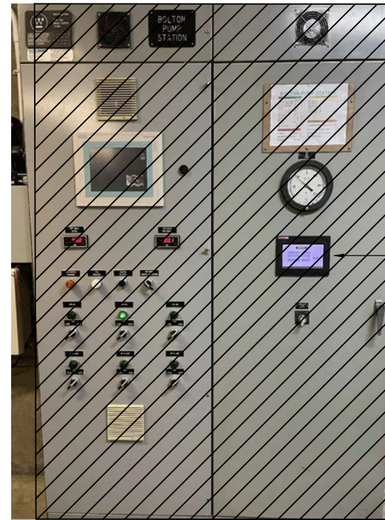
EXISTING CONTROL PANEL AND BUBBLER SYSTEM DEMOLITION ②
