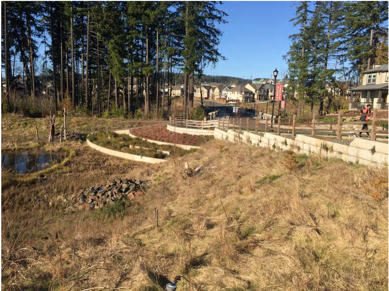
River Terrace Regional Stormwater Facility, Tigard
