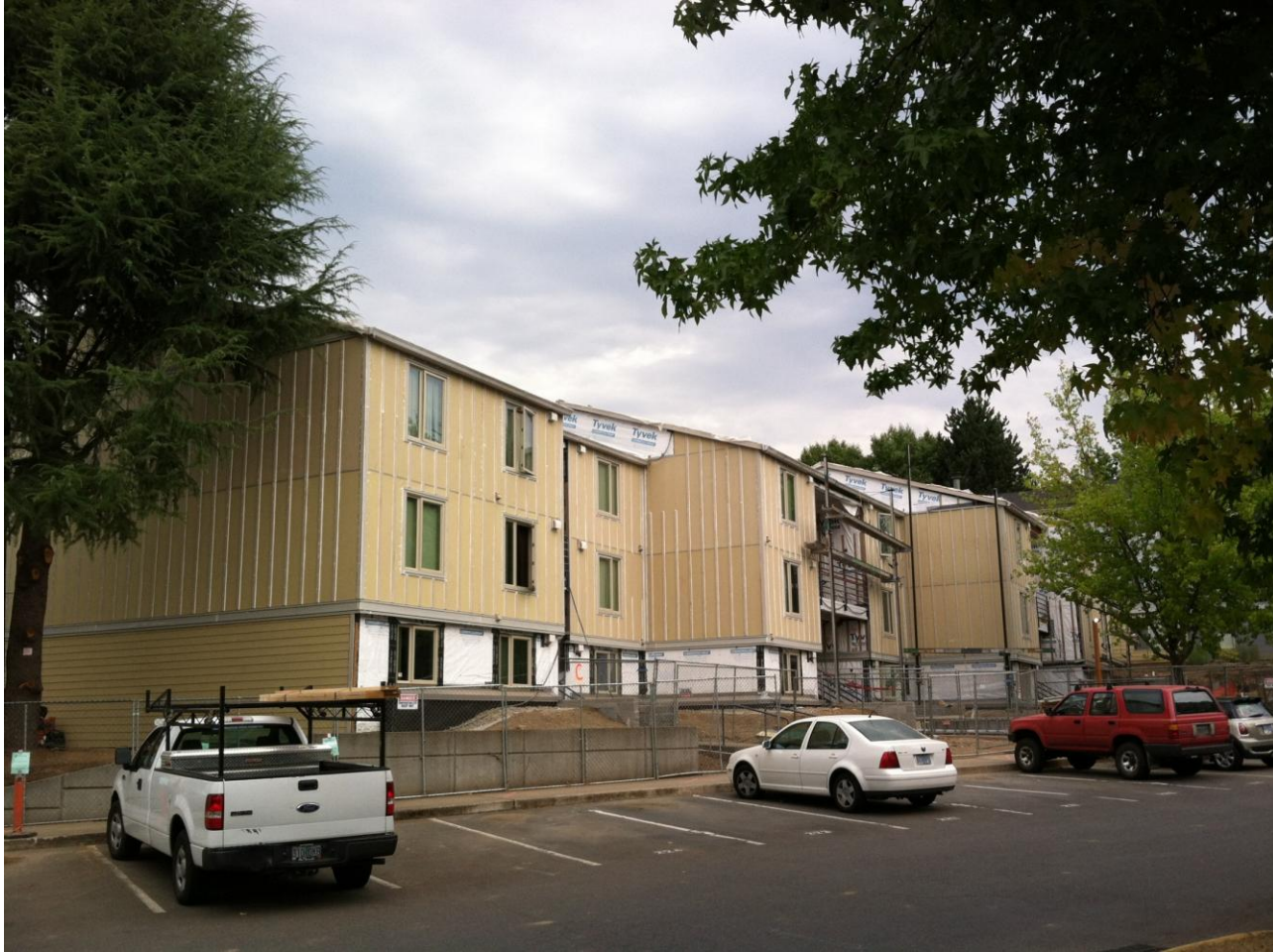
Siding in progress.
