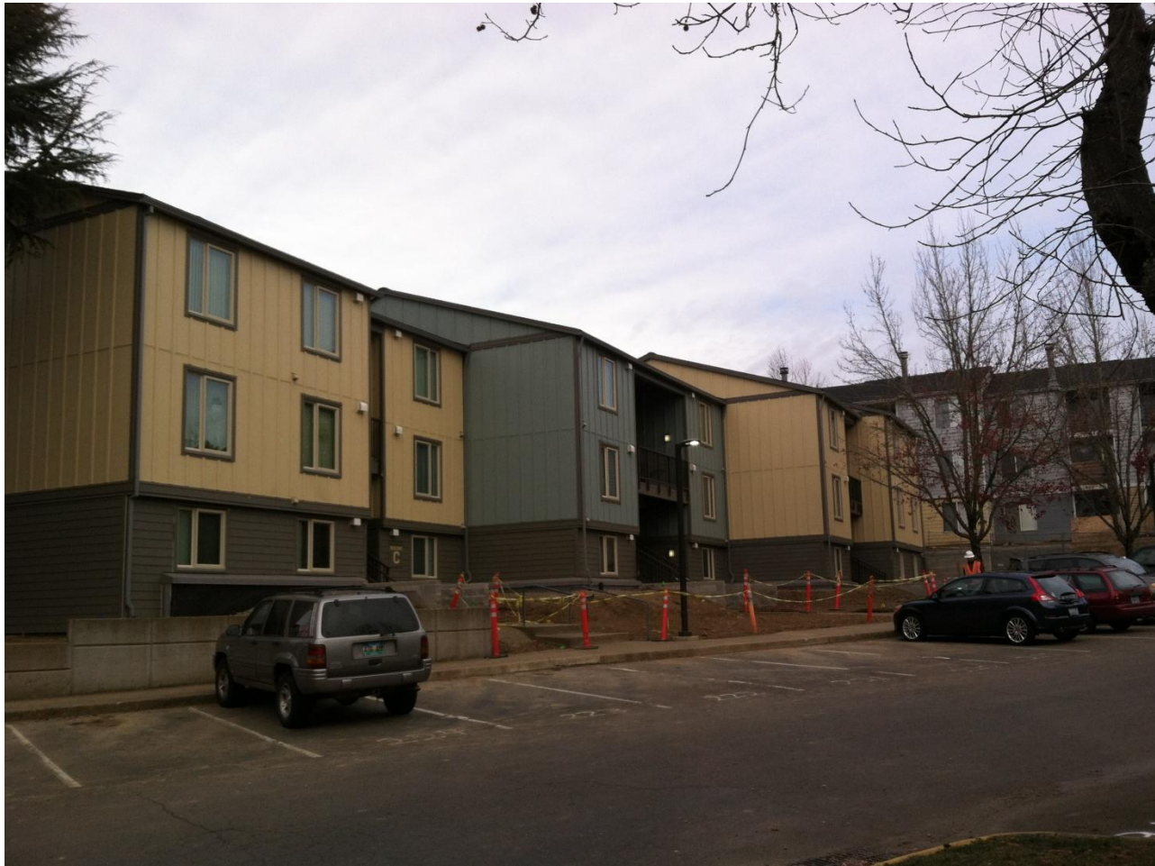
Building C complete.
