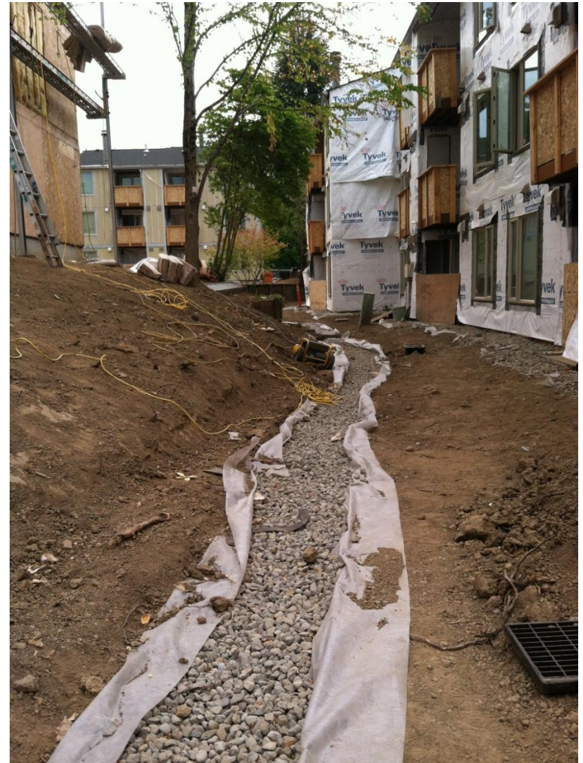
New site drainage
