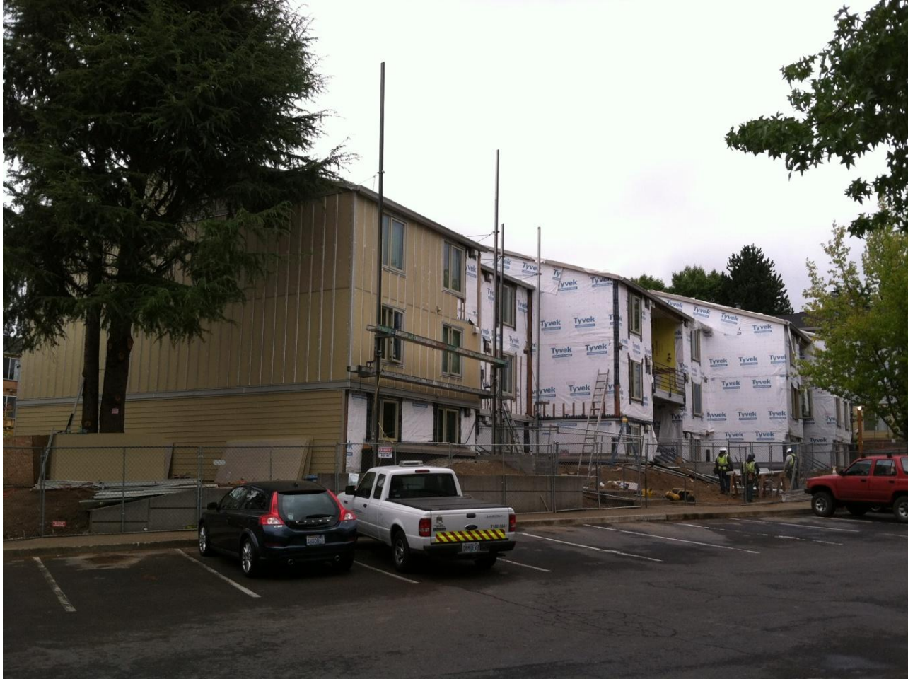
Siding getting underway.
