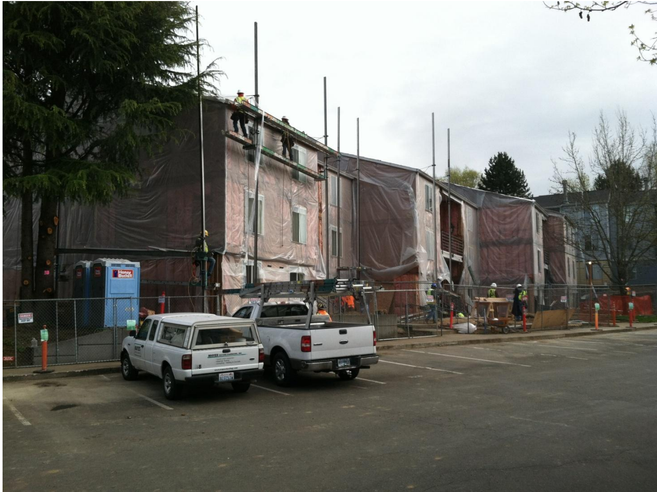
Structural repairs and remediation work underway.
