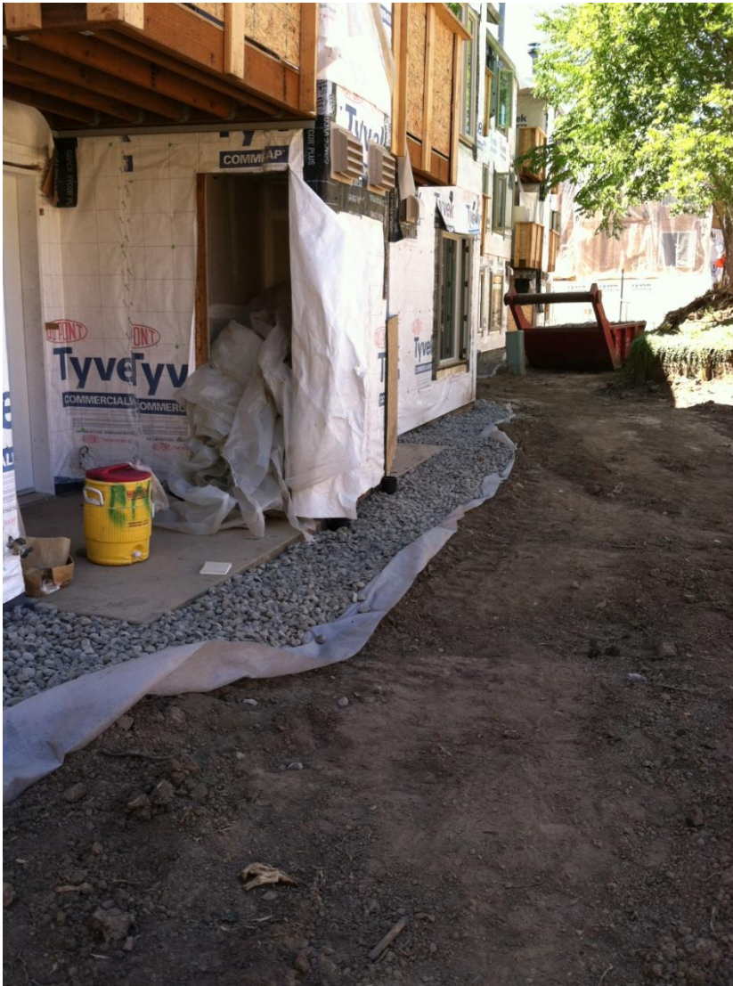
New foundation drainage
