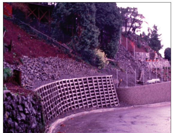
Retaining wall at bottom of a slope. Photo credit: Scott Burns.
