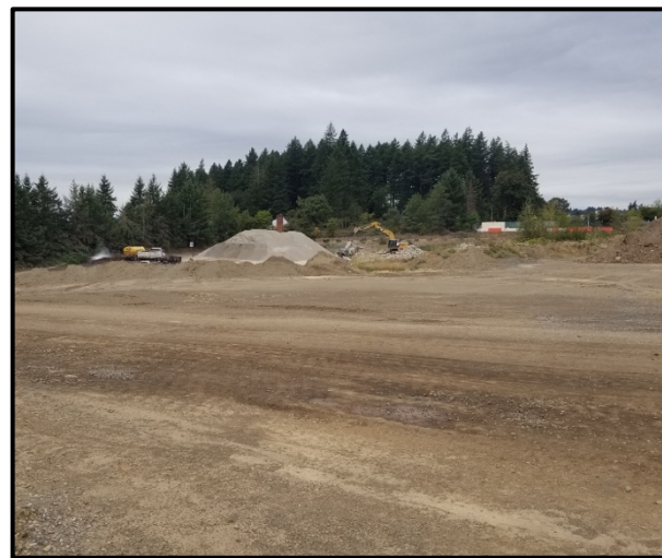
View of site with fill piles and equipment
