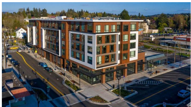
Test case/opportunity site near Park Ave. light rail station ≈ 100 units/acre
