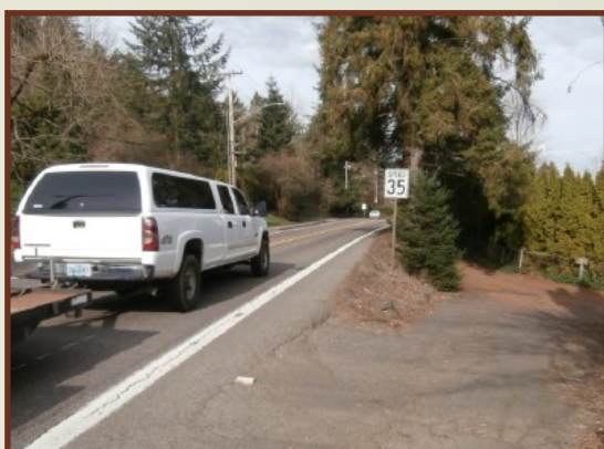
Existing conditions provide limited shoulder in multiple areas within project boundary
