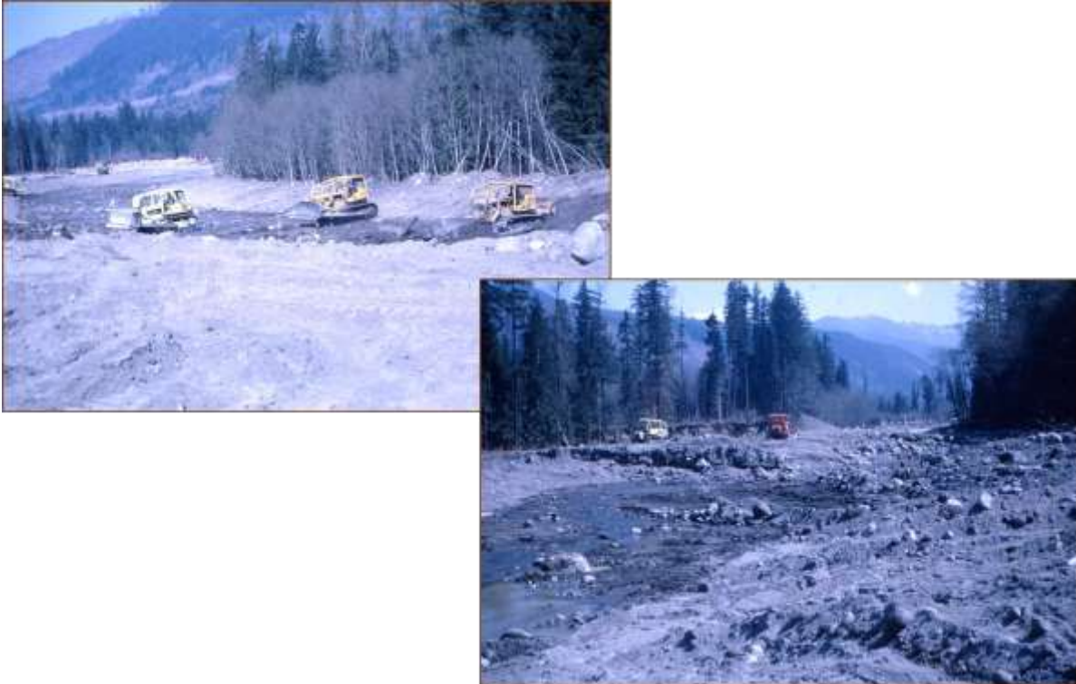
Figure 19. Army Corps of Engineers Bull Dozers Re-Grading the 1964 Channel. Following the 1964 flood the ACOE mechanically graded over the active channel to recover the pre-'64 single stem channel. The re-grading straightened and shortened the 1964 channel, increasing the channel gradient in the process. Note the large proportion of fine grained materials comprising the flood deposits. Photos courtesy of Raymond Arrigotti.
