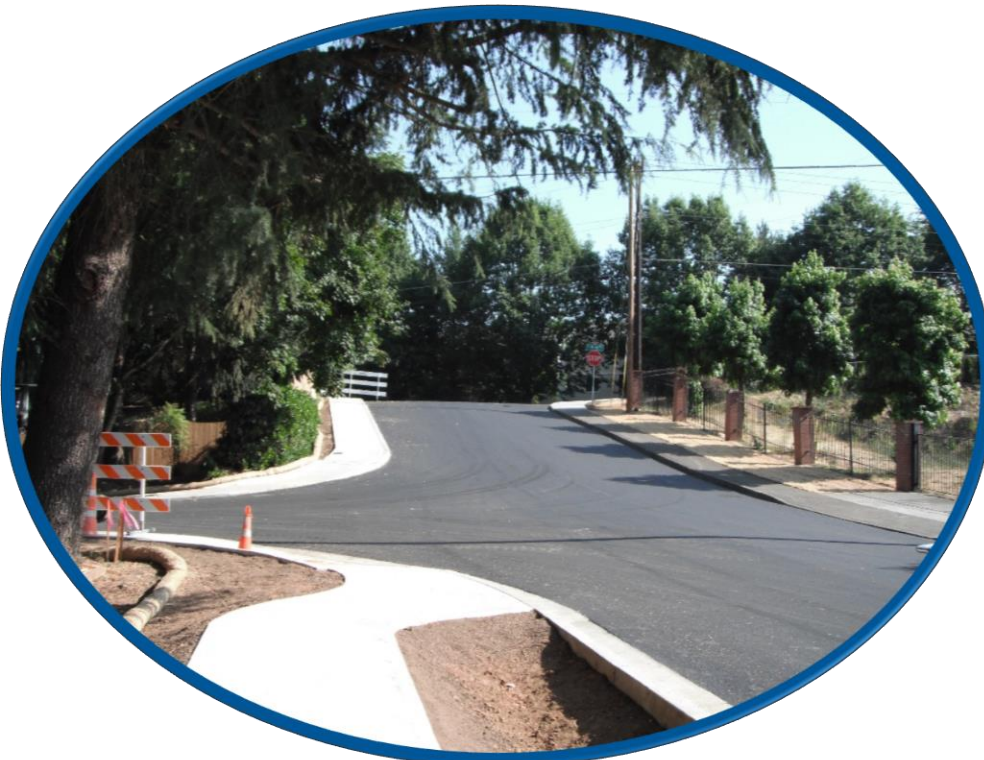
70 th Avenue improvements included paving, curb, sidewalk on one side and drainage.
