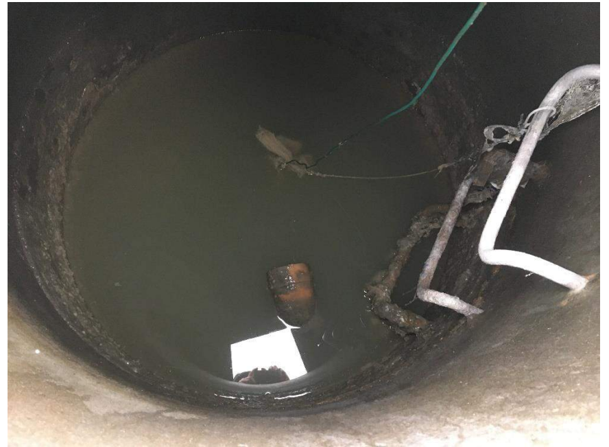
Diversion Structure Interior
