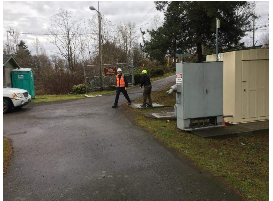
WRRF Entrance and Influent Pump Station
