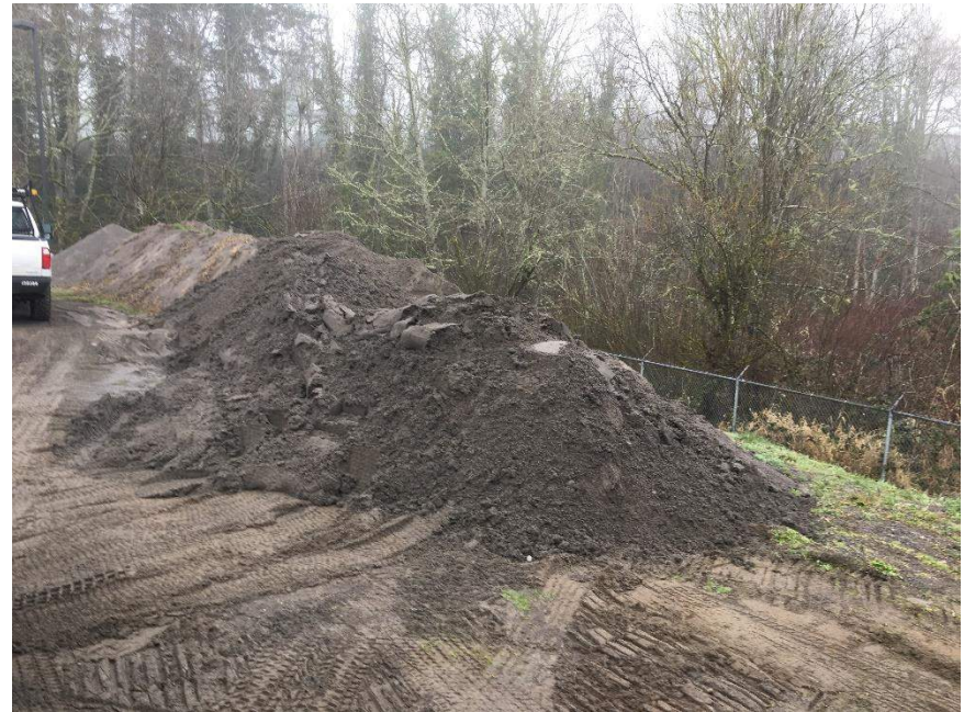
Onsite Sand Stockpile
