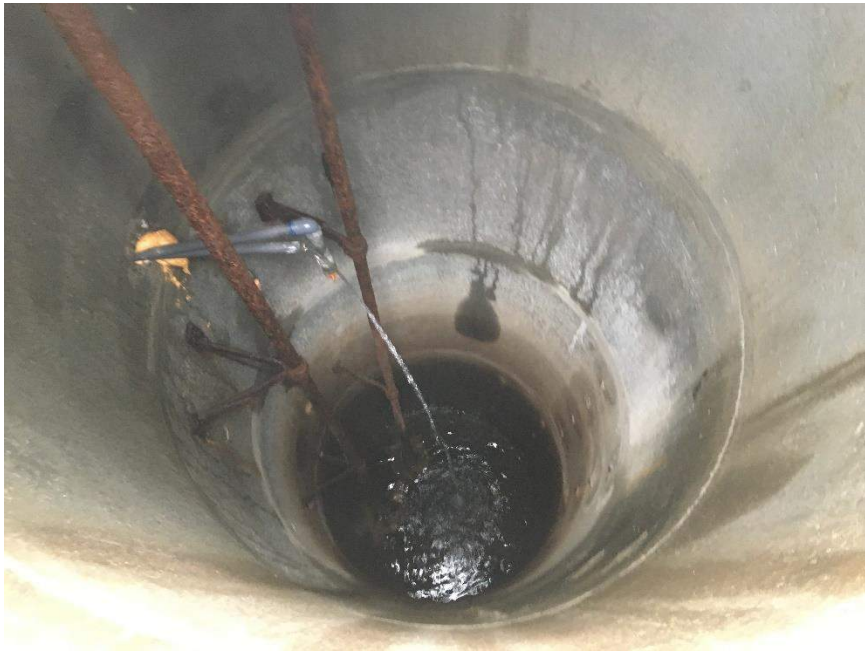
Chlorination Manhole Interior
