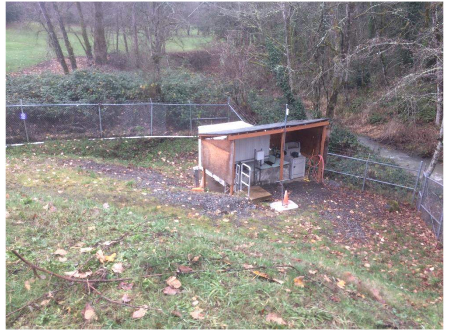
Disinfection & Effluent Shed
