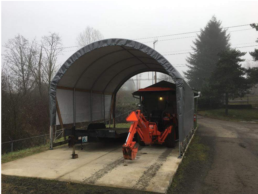
Equipment Storage Pad and Cover
