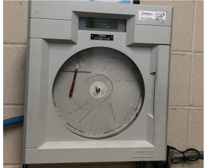
Influent Flow Meter
