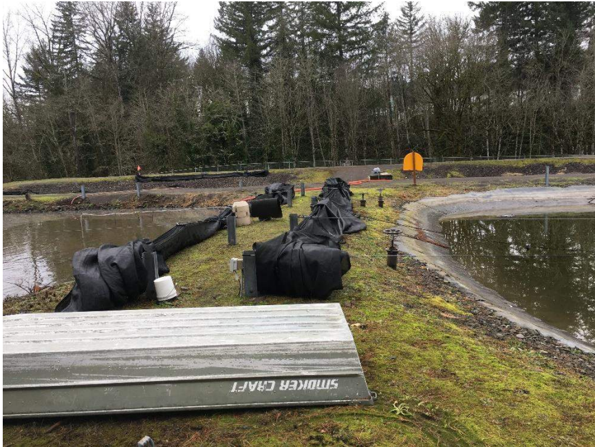
Aeration Basin Covers
