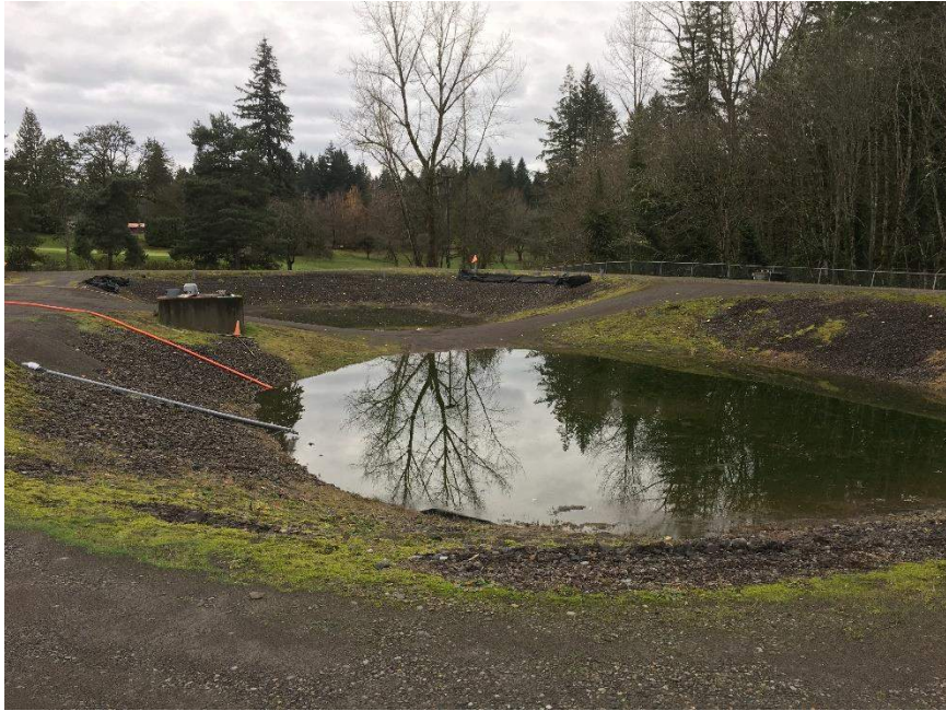
Splitter Box and Sand Filters
