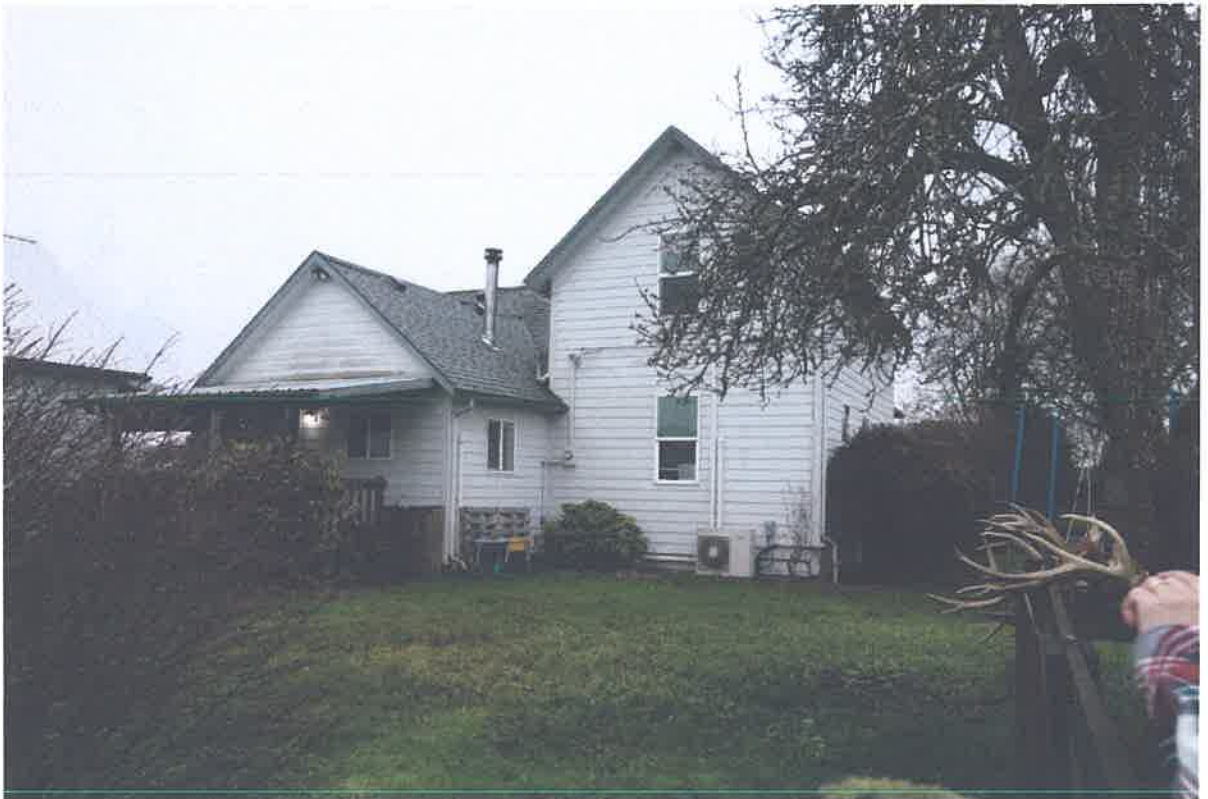
Figure 5. North side of house, taken on December 11, 2019.
