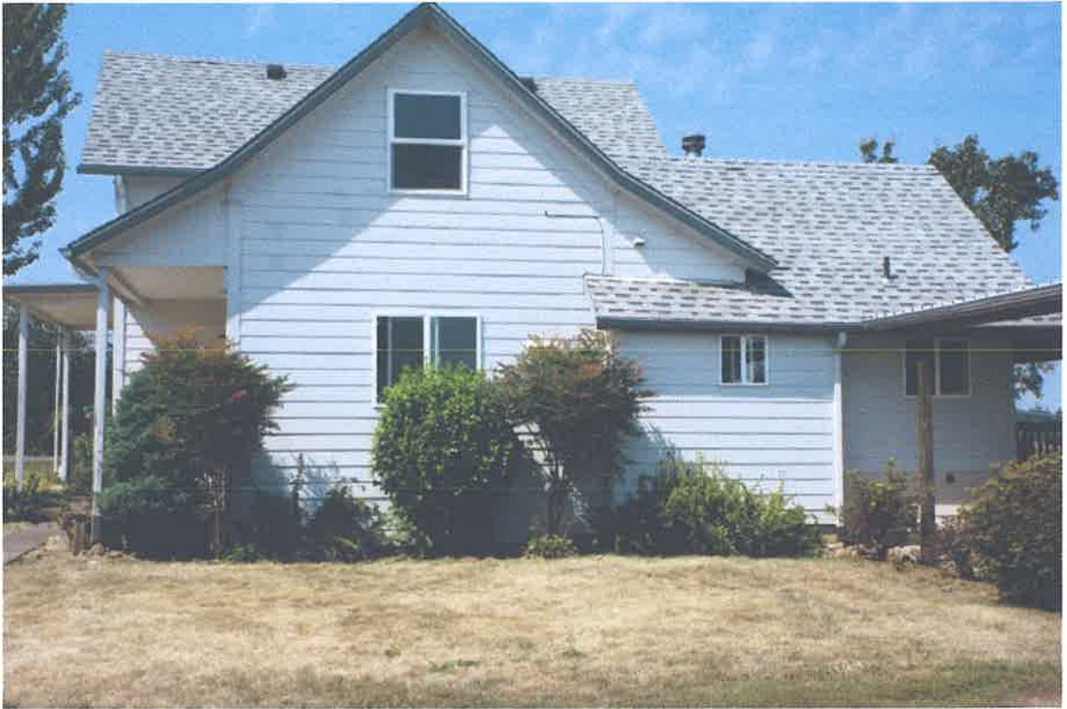
Figure 4. East side of house, taken on August 14, 2014.
