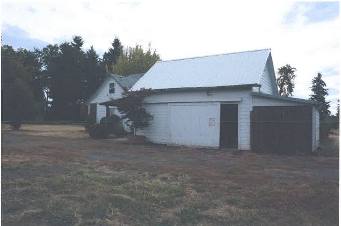
Figure 9. East side of woodshed/garage with house in the background, taken on August 14, 2014.
