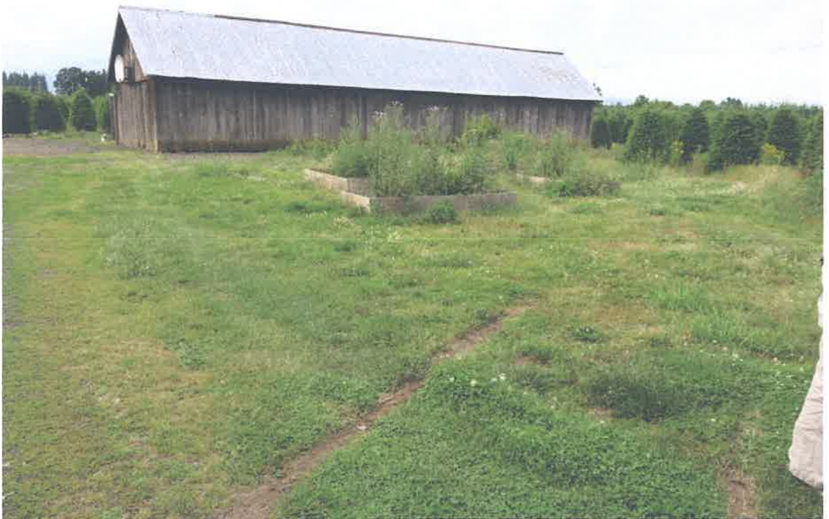
Figure 10. South side of machine shed, taken on June 25, 2014.
