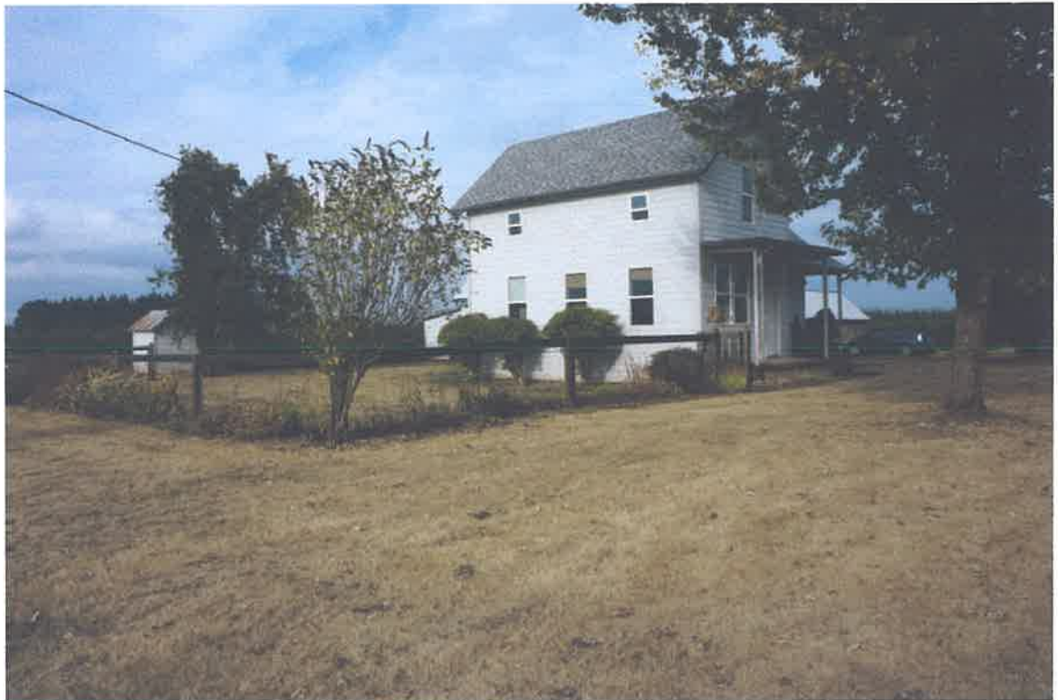
Figure 7. Southwest corner of house, taken on August 14, 2014.
