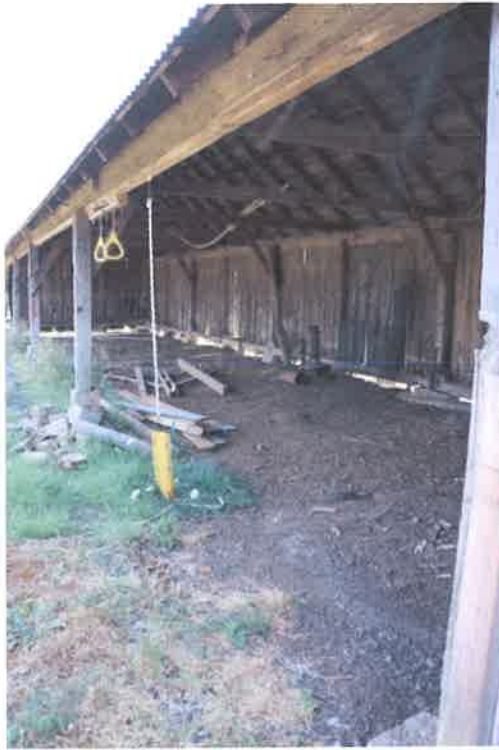
North side of machine shed
