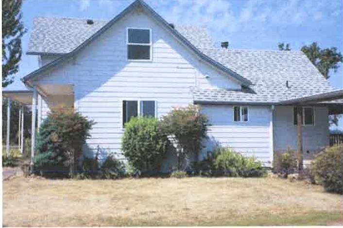
Photographs of existing home/farm complex, taken August 24, 2014 East side of house
