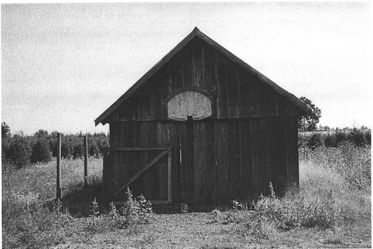
Figure 11. West side of machine shed, taken on August 14, 2014.
