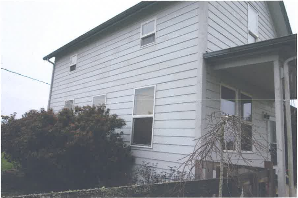
Figure 8. West side of house, taken on December 11, 2019.
