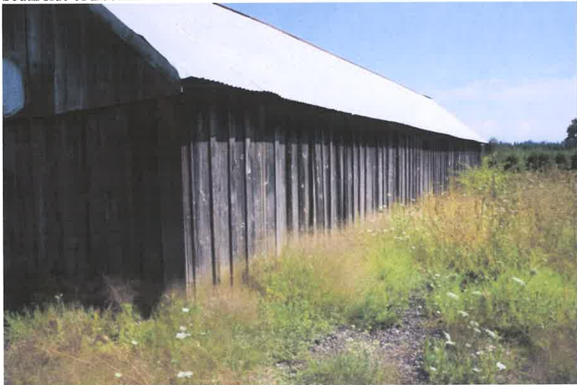
South side of machine shed
