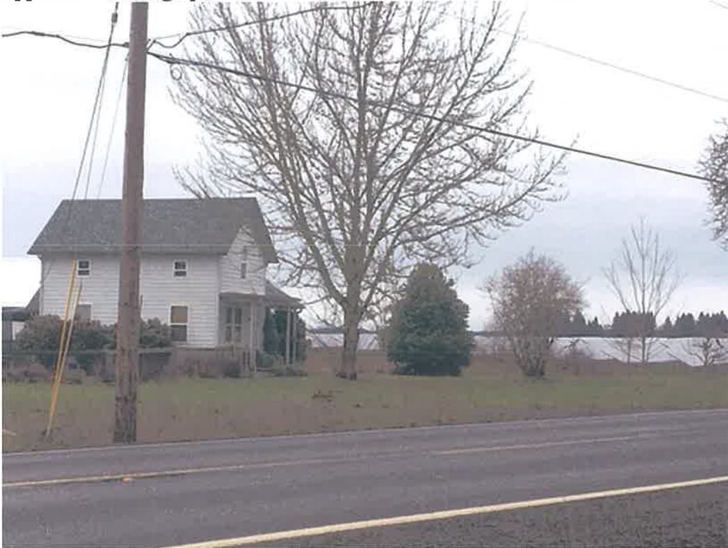
Figure 2. House from west side showing solar panels on the 12-acre parcel to the east, taken on January 22, 2020.
