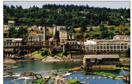
The former Blue Heron Paper Mill represents a truly unique development opportunity that would create a landmark destination for the state.
