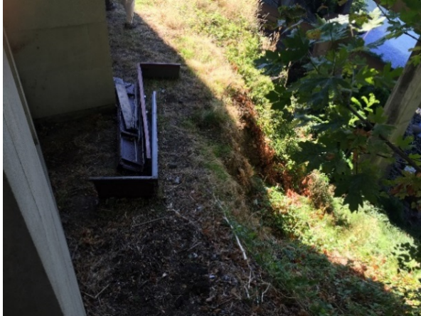
Cliff at Willamette River (looking south)
